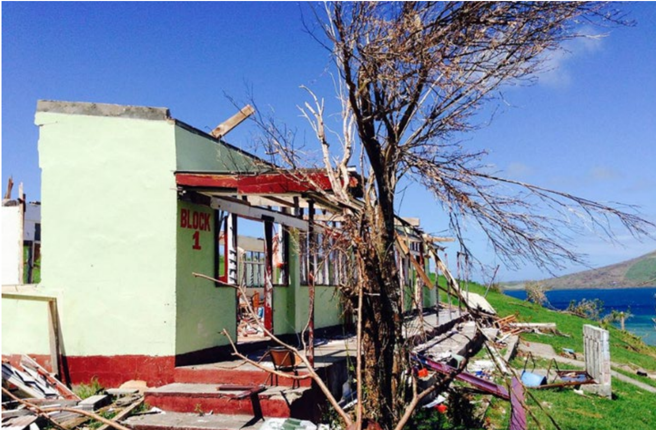
Photo 12: Damage from Cyclone Winston, Fiji
