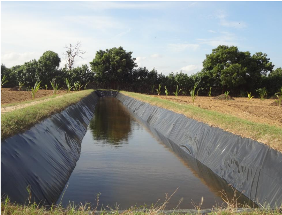
Low cost rain water storage model. Photo credit: Paramanathapillai Seran
