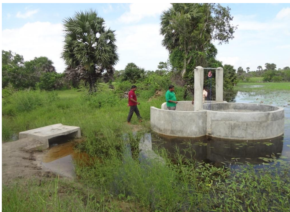
Flood proof dug well. Photo credit: Paramanathapillai Seran
