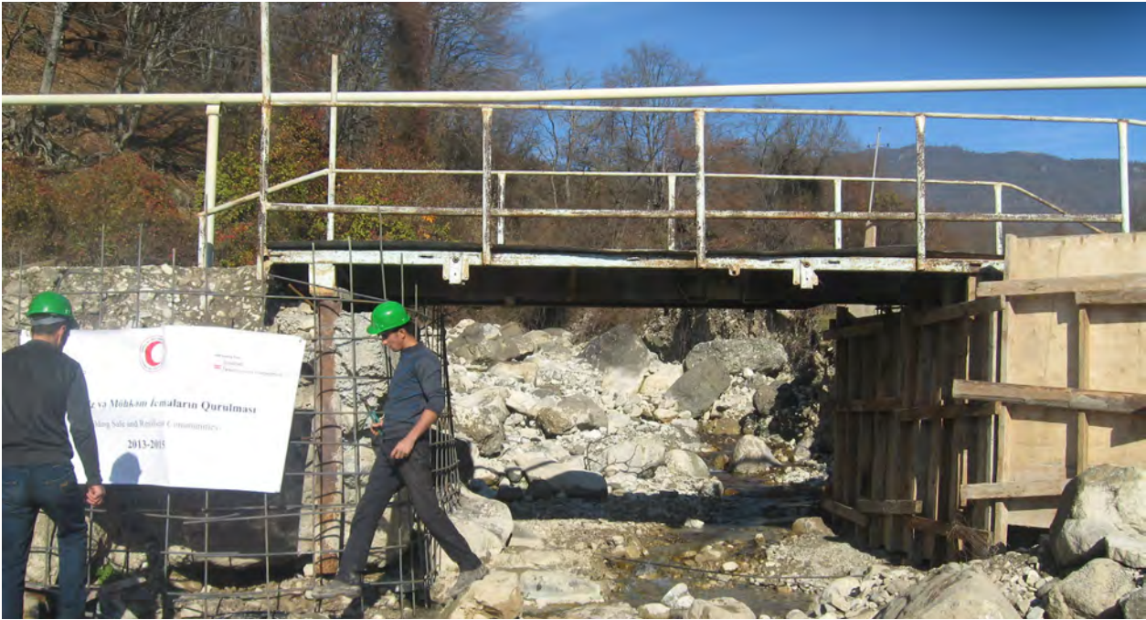
Bridge repair Diyalli Azerbaijan.
