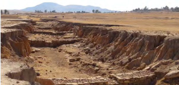
Gully erosion control structures (Source: WFP).
