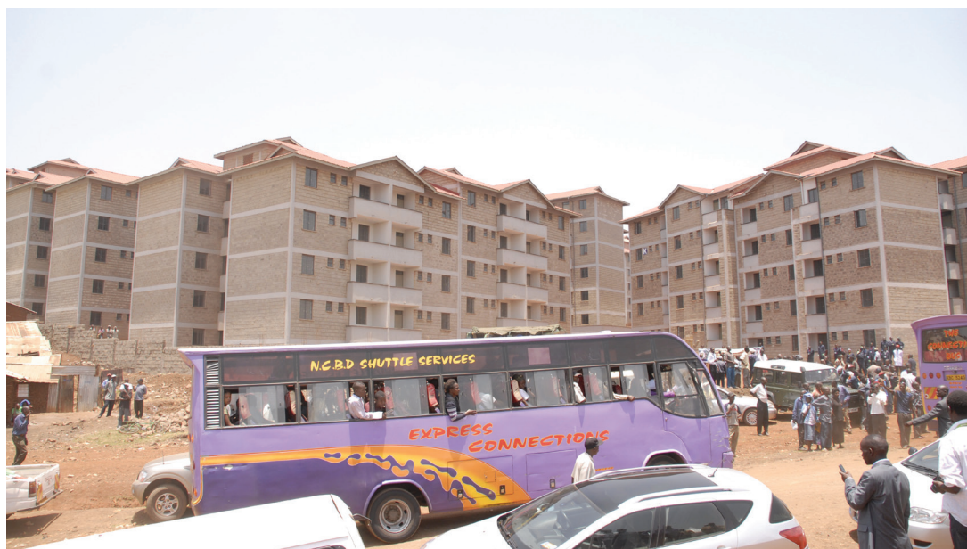
Slum upgrading project in Kibera-Nairobi, Kenya © UN-Habitat
