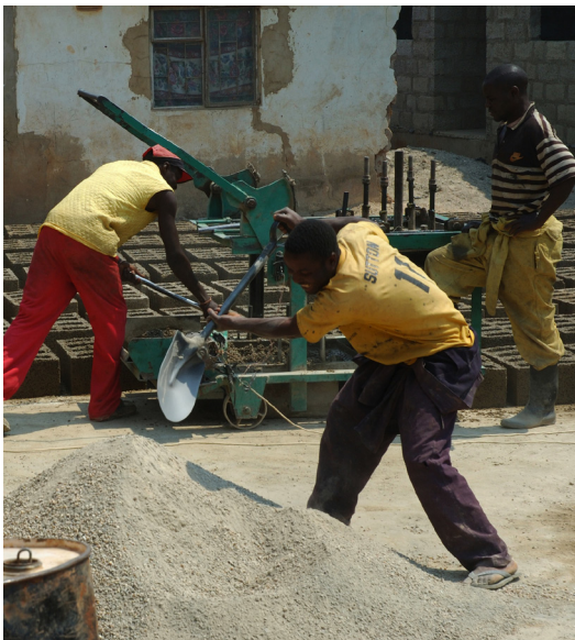
Construction in Zambia © UN-Habitat
