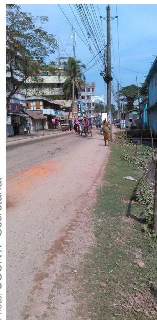
Open sewage alongside the road in Patuakhali, Bangladesh Figure.
