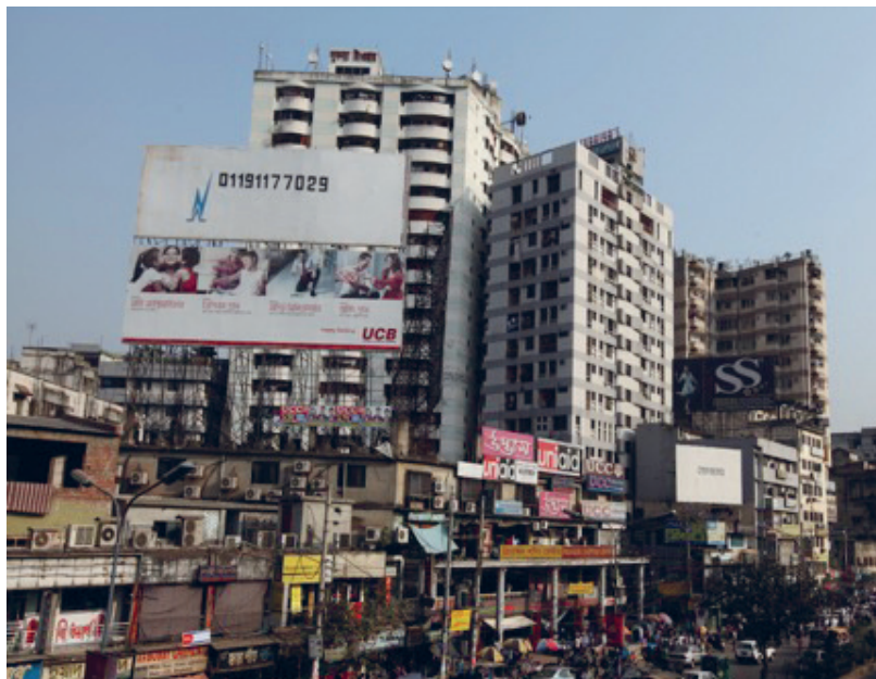
The number of high rise and modern buildings has been growing in Dhaka thus increasing exposure to physical risks.
