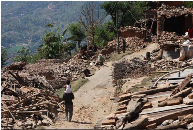
Nepal Earthquake Affected Village in Karve District.
