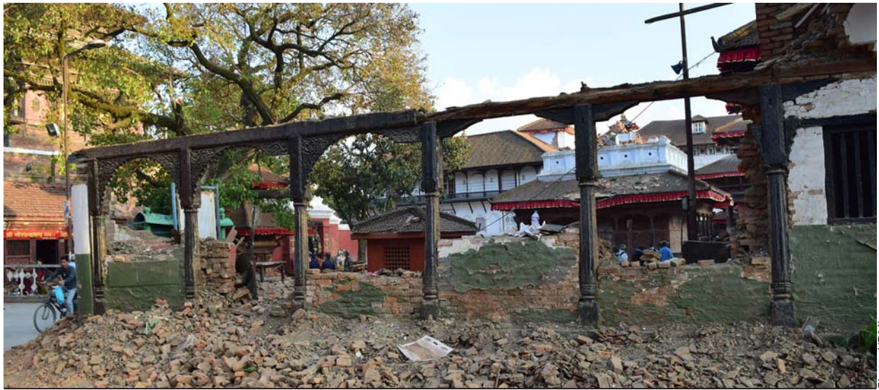
The damaged Basantpur square (Kathmandu) after the earthquake.
