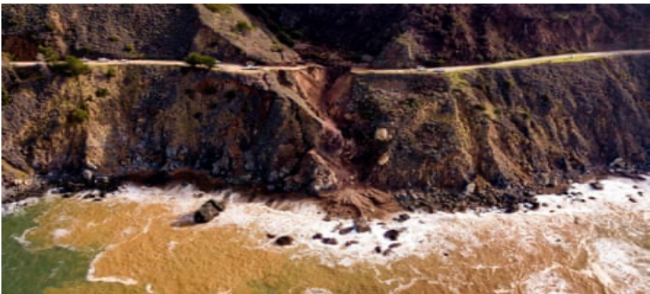
Figure 2: Landslide causing a 150ft section of Highway 1 to wash away into the sea. Source
