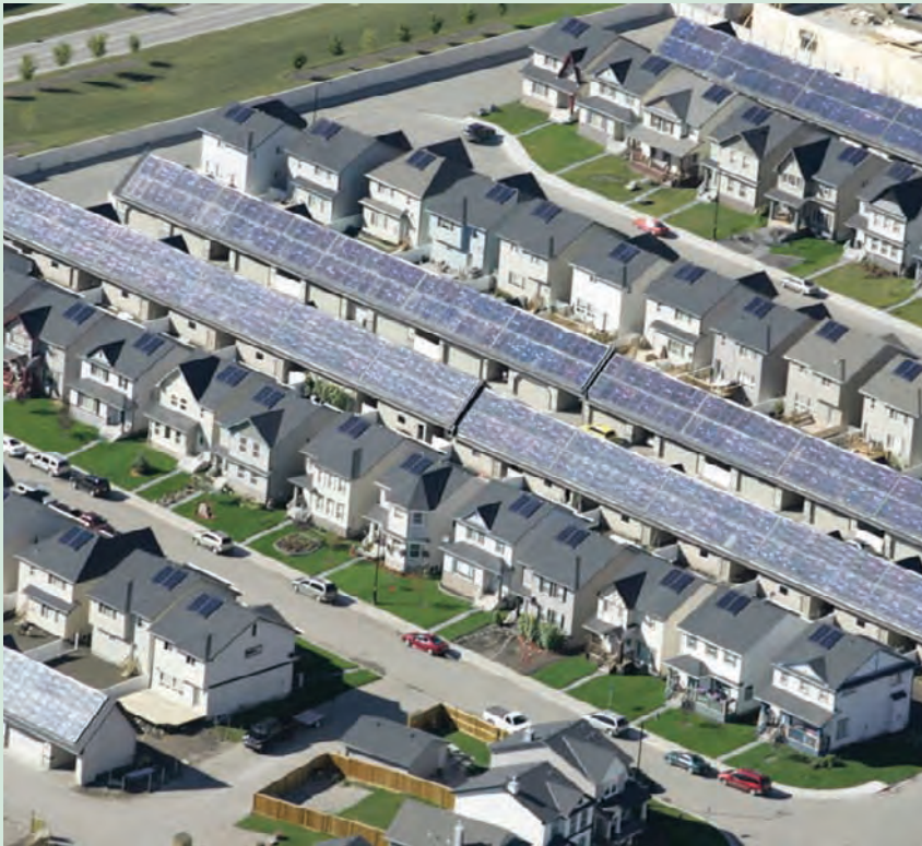
Figure E-17: Aerial view of the 52-home Drake Landing Solar Community, 2007 (Natural Resources Canada, 2007. Reproduced with the permission of the Minister of Natural Resources of Canada, 2012)
