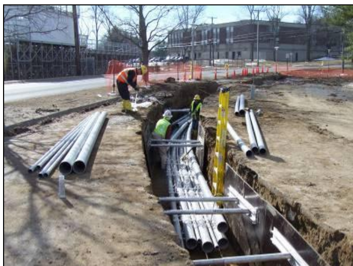
Figure 15 - Underground Distribution Conduit Installation
