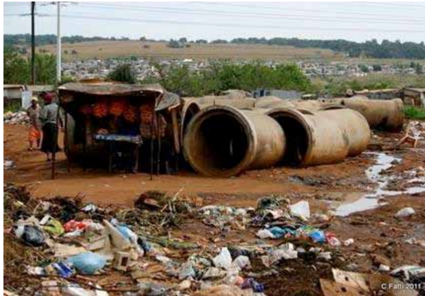
Illustration 2: Abandoned storm water pipes in Tembisa from uncompleted storm water system, abandoned due to resistance from community to move (Photograph courtesy of Christina Fatti).
