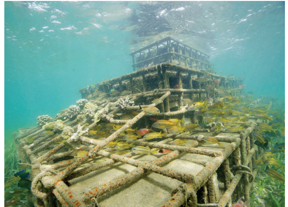
Coral reef growth on the breakwater structure one year after implementation, in 2015. The structures are designed to restore the wave-breaking function of the reef, and therefore reduce wave energy reaching the shore, which typically exacerbates coastal erosion and flooding. (Photo by Tim Calver.)
