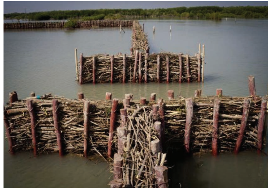
Permeable barrier to trap sediment. (Photo by Nanang Sujana for Wetlands International.)
