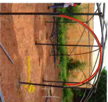
Arches to improve the structural resistance between poles
