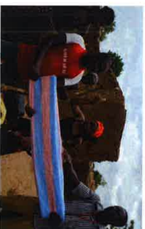
Physical barrier to avoid water from the ground inside the shelterproofing
