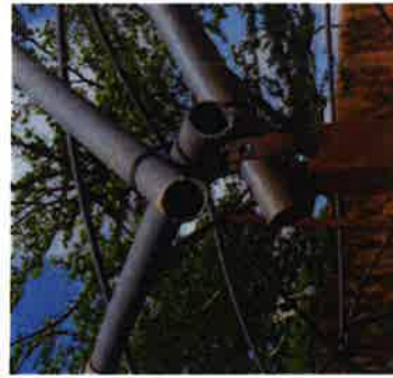
Metallic wire for connections cut and attached with pliers
