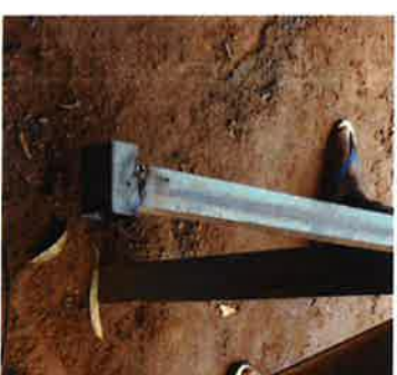
Metallic piece on the foot of the pole – improving resistance in soft soil
