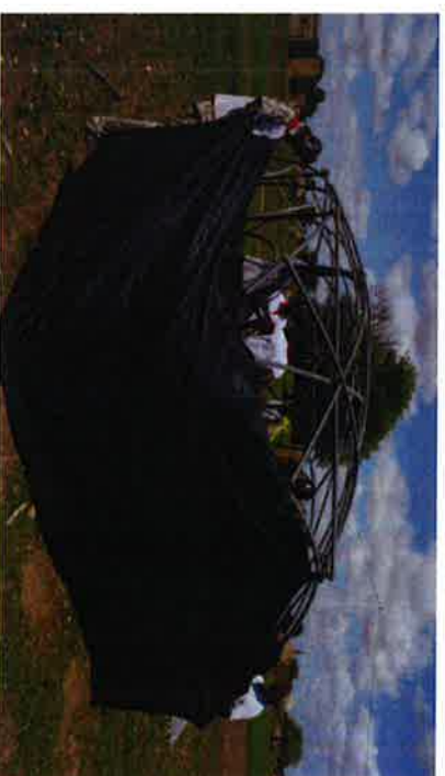
"Warehouse" version with walls in double layer of shade net
