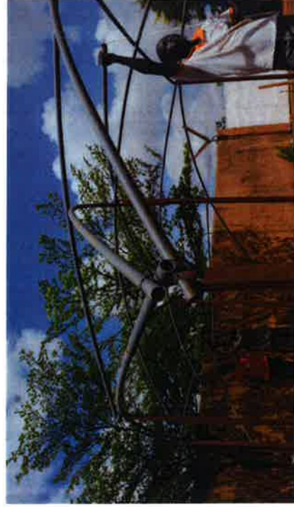
Double curved surface increases rigidity in all directions
