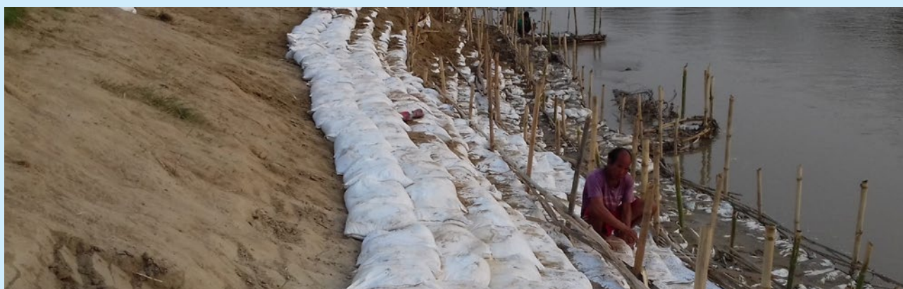
Photo: Bio-dyke construction work at Bangalipur, Bardiya Source: Practical Action, 2021
