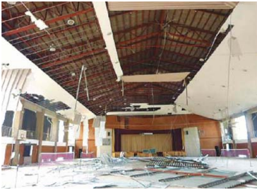
Figure 2.8 Fallen ceiling panels in school gymnasium
