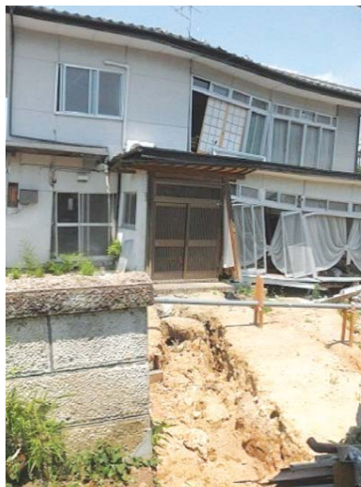
Figure 2.10 Houses damaged by failure of retaining walls
