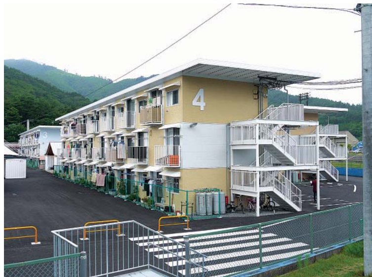
Figure 22.6 Multiple-story temporary housing made with stacked containers
