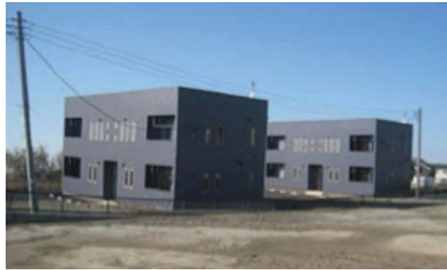
Figure 2.9 Subsidence of houses from liquefaction
