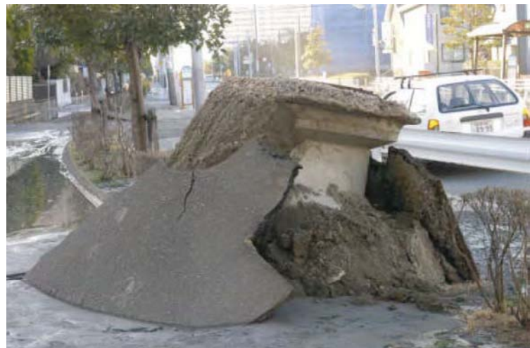
Figure 20.3 Manhole raised by liquefaction in Urayasu City
