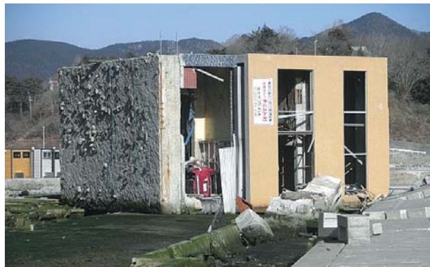
Figure 2.5 Reinforced concrete building damaged by buoyancy
