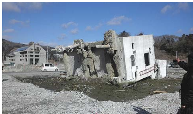
Figure 2.7 Overturned building of reinforced concrete with pile foundation
