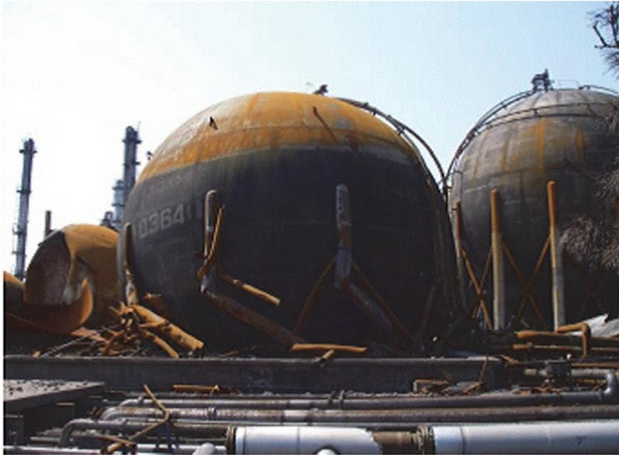
FIGURE 2.3 The Refinery's Tank 364 That Collapsed During the Earthquake
