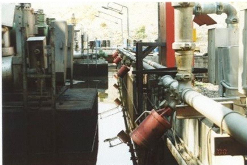
FIGURE 2.2 New Foam Spraying System Secured Along a Reinforced Concrete Containment Dike
