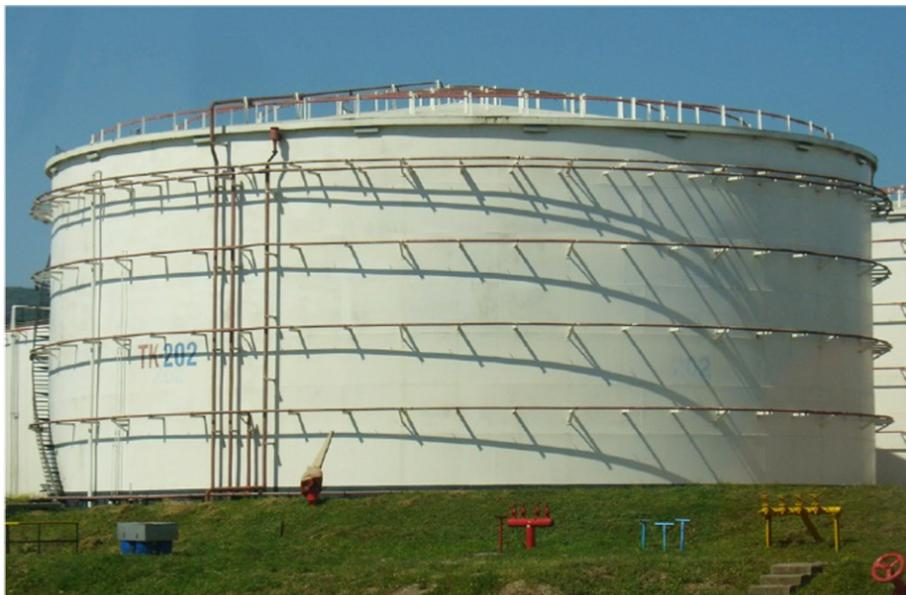
FIGURE 13.7 Retrofitting of a Storage Tank Affected by the 1999 Kocaeli Earthquake in Turkey With a Sophisticated Sprinkler System
