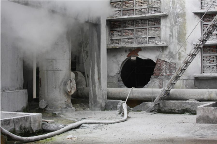
FIGURE 13.8 Damaged Retention Wall During the 2008 Wenchuan Earthquake
