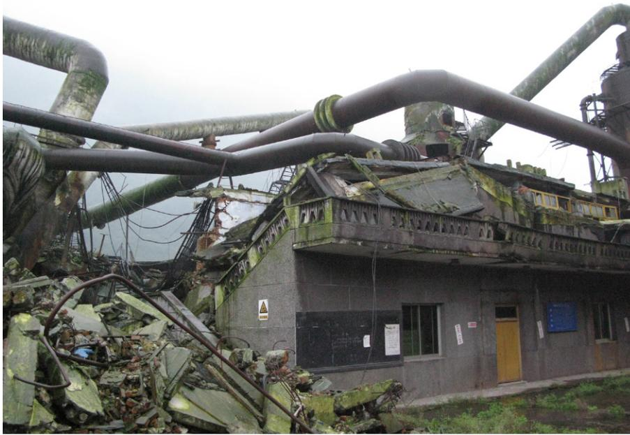
FIGURE 13.1 Pipes Collapsed Onto a Building at a Fertilizer Plant During the 2008 Wenchuan Earthquake in China
