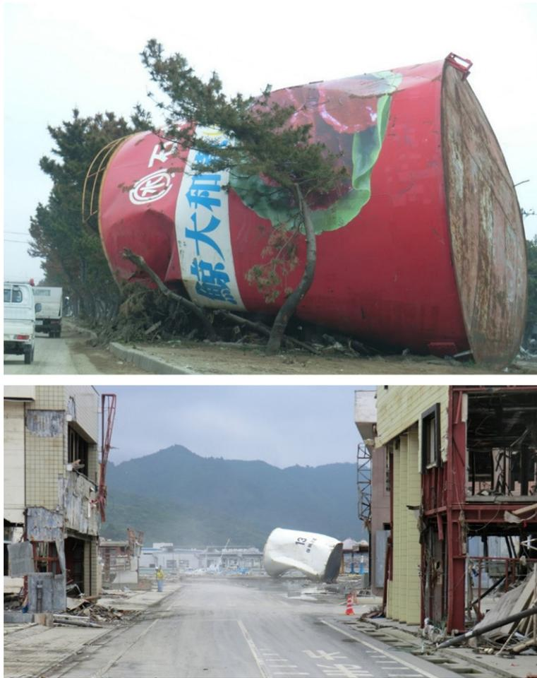
FIGURE 13.5 Examples of Damage to Oil Storage Tanks in Miyagi Prefecture During the Great East Japan Tsunami in 2011
