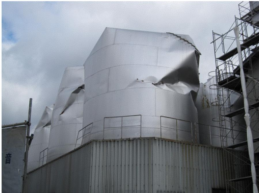
FIGURE 3.1 Diamond Buckling of Silos Near the Epicenter of the 2011 Tohoku Earthquake in Japan
