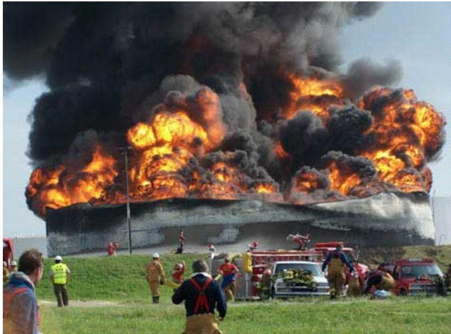
FIGURE 3.9 Lightning-Triggered Fire in a Gasoline Storage Tank in Oklahoma
