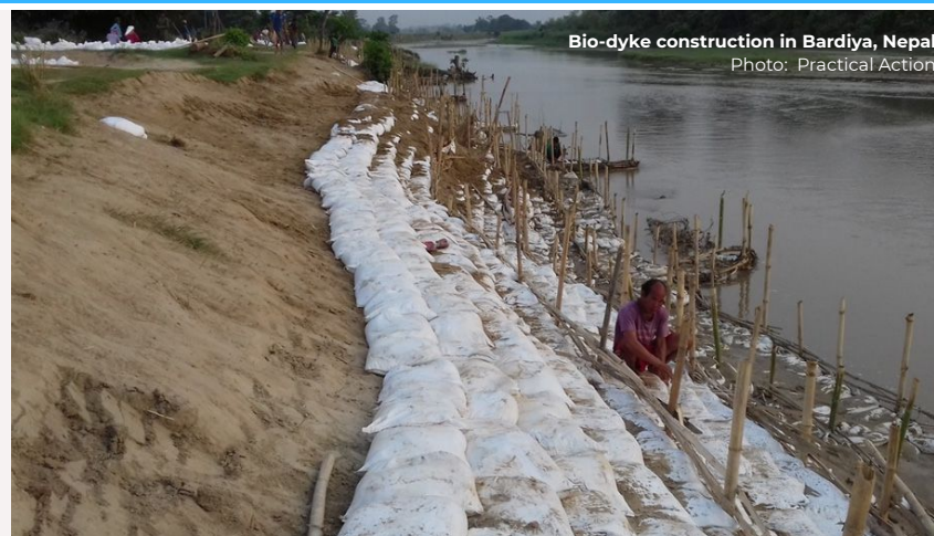
Fully developed bio-dyke Photo: Practical Action
