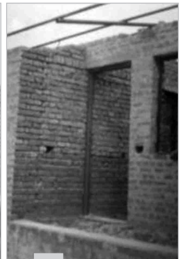
Figure 3.10: Brick building under construction
