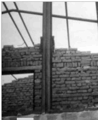
Figure 3.11: Pre Cast RCC lintel above the opening
