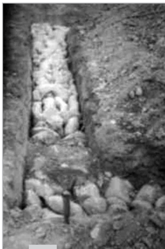
Figure 3.8: Stone Masonry in Foundation
