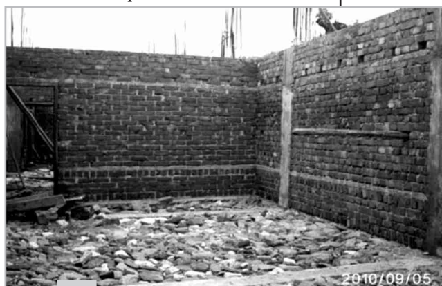
Figure 4.10: Constructing Sill and Lintel bands has become popular in Dharan
