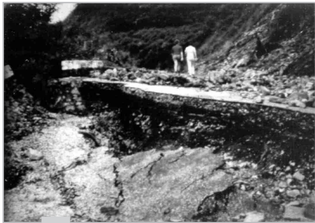
Figure 3.4: The damage of road in Koshi Highway
