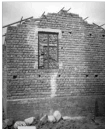
Figure 3.13: Detached toilet blocks for the houses
