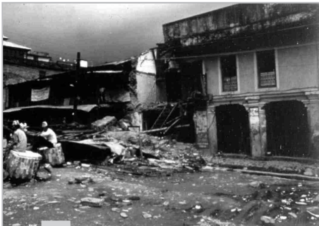
Figure 3.3: Building damage in Naya Bazar of Dharan
