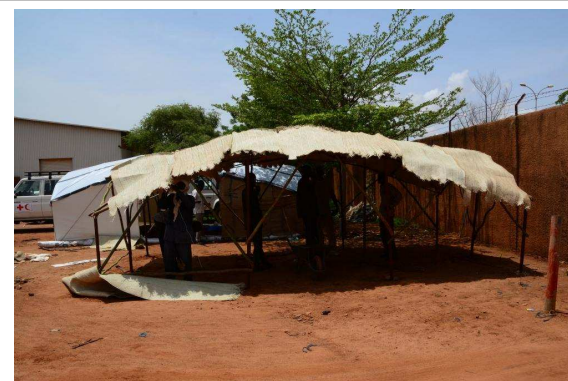
Vegetal mats as a first layer of the dome
