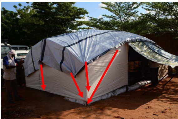
Quality plastic sheeting fixed to the bottom part of the metallic poles
