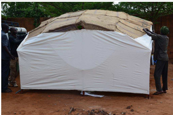
Jute bags stitched over the dome structure
