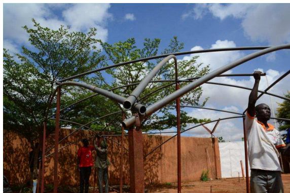
Metallic wire for the unions attached with a clipper
