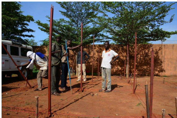
The central pillars are higher to increase the inner space
