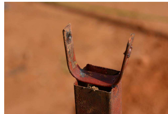
U-piece on the head of the pillars to ensure the union with the arch
