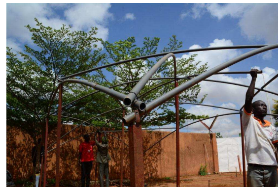
Double curved surface increases resistance in all directions
