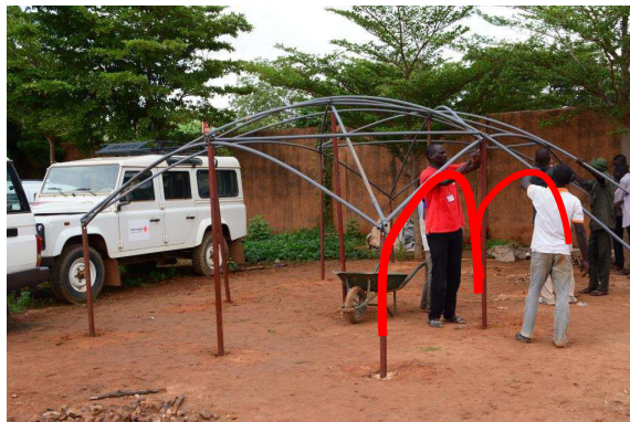
Arches to improve the structural resistance between pillars
