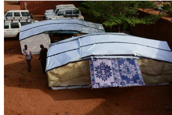
Shelters with the same structure concept but alternative cladding materials
