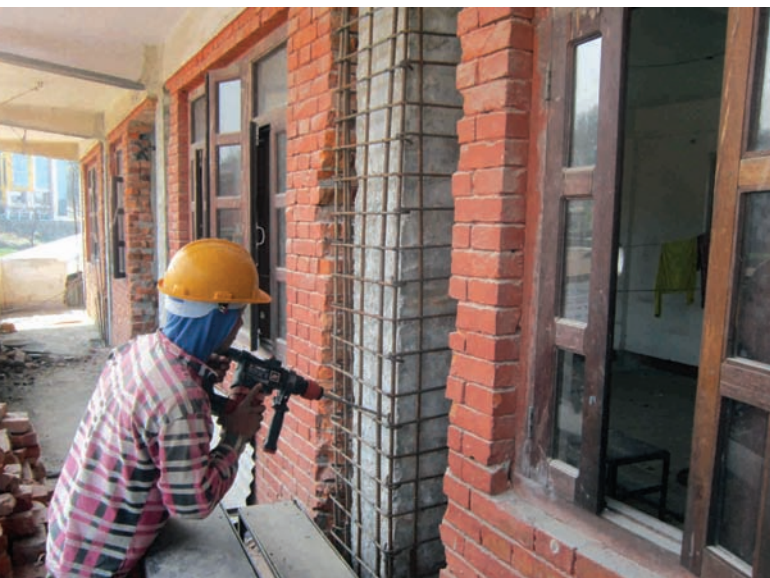
Fig2: Retrofitting of Adarsha Aajad Secondary School
