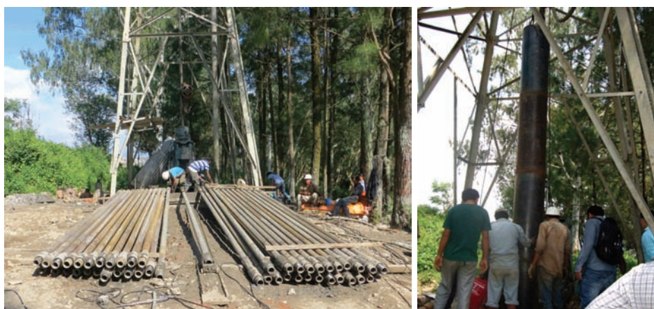
Fig.12: Deep tube well construction at TU, Kirtipur
