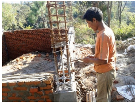
Fig.13: Generator house construction at TU, Kirtipur
