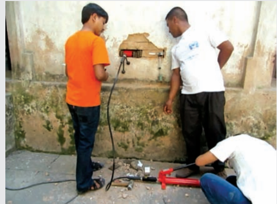
Fig3: Conducting shear test at Kaiser Mahal
