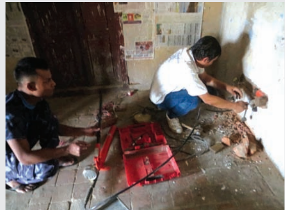
Fig5: Conducting shear test at Charkhal building
