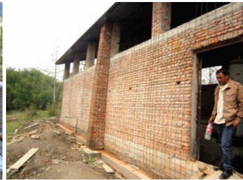
Fig.14: Retrofit of water treatment plant building at TU, Kirtipur
