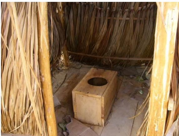
Pit latrine (not ventilated)
