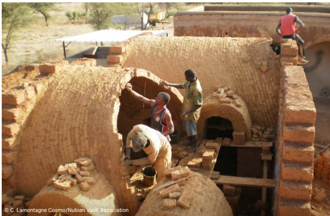
Four men working on the construction of a Nubian vault.
