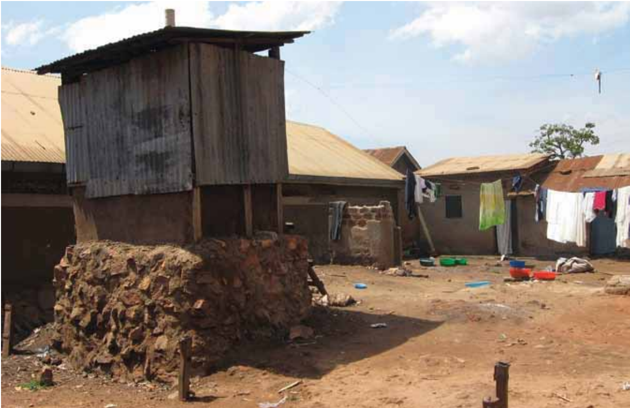
▲ This type of pit latrine is quite common in Kampala's slum areas. The toilet slab is elevated to protect it against flooding, which happens regularly. ©SuSanA Secretariat. Licensed under the Creative Commons Attribution 2.0 Generic license.
