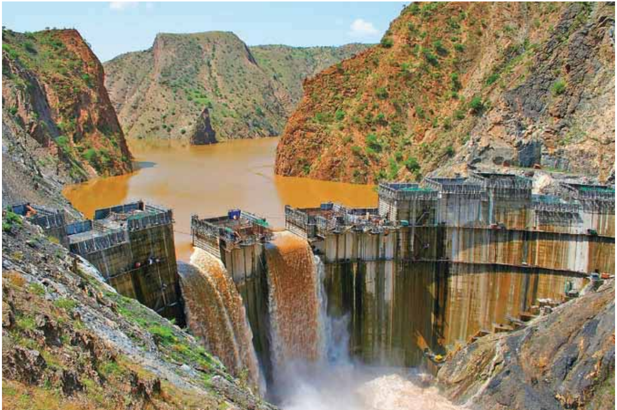
▲ The Tekezé Dam is a double-curvature arch dam in the Tigray region of northern Ethiopia on the Tekezé River, a Nile tributary that flows through one of the deepest canyons in the world. The dam consists of four turbines, together generating 300 MW. ©Paul Snook
