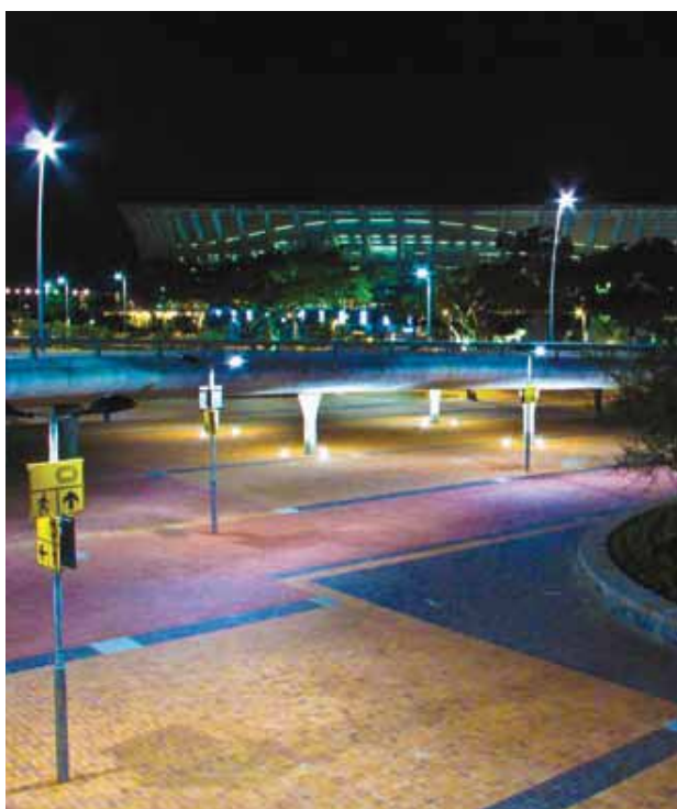
▲ The pedestrianised 'Fan Walk' approach to Greenpoint Stadium, Cape Town. The maintenance of new infrastructure for the 2010 World Cup has added an extra burden on local government.
