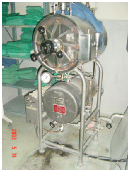
Photo 5: Autoclave machine without anchorage.
