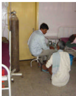
Photo 11: Un-hooked oxygen cylinders may fall over.
