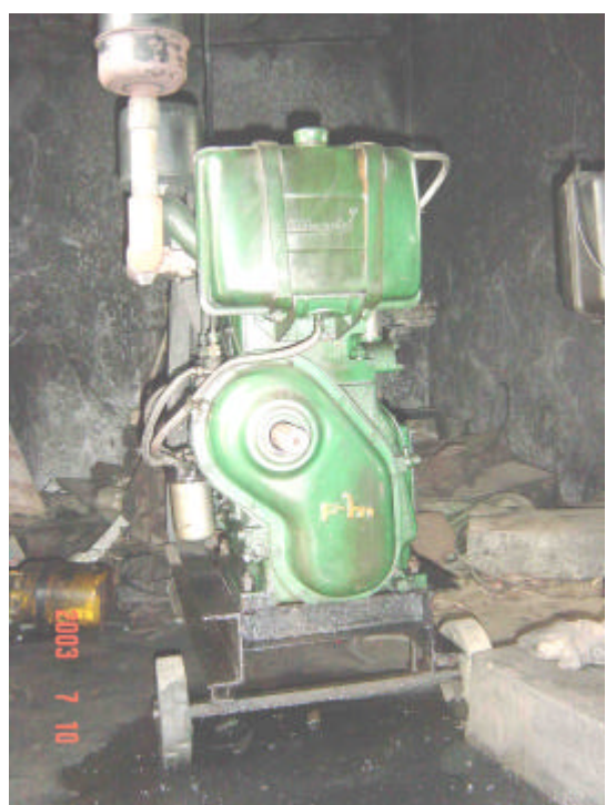
Photo 4: A generator on rollers can slide and overturn in an earthquake causing functional loss.
