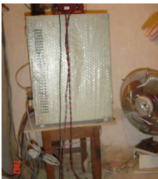
Photo 7: Communication equipment on a temporary type stand. It needs a proper stand with anchorage and fixing.
