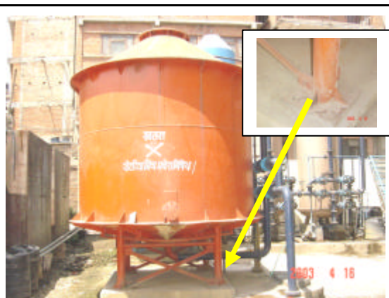
Photo 6: Water treatment tank which has a provision for bolting at the base but was found not bolted.
