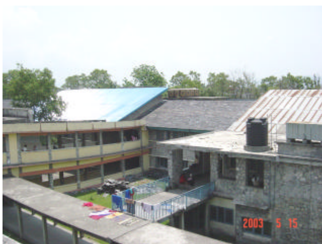
Photo 1: Buildings of different height, shape and structural properties connected with each other can cause severe pounding during earthquakes.
