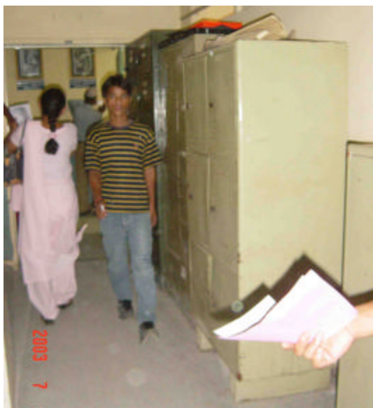
Photo 3: These cupboards can block the corridor and are a life safety hazard.
