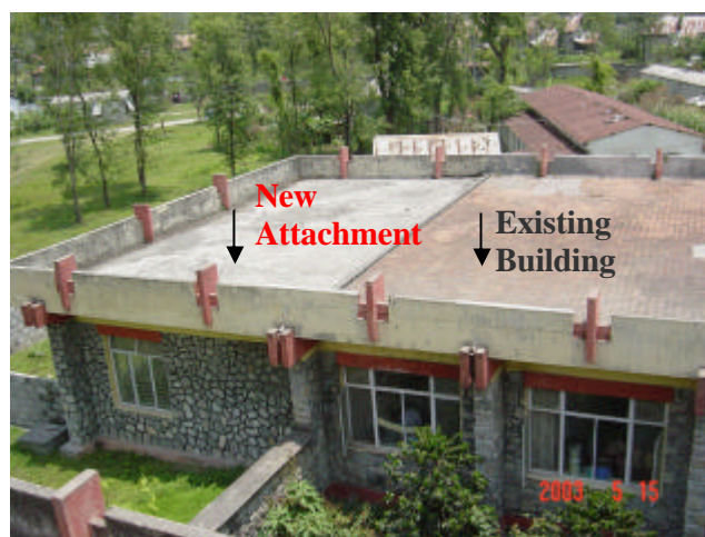
Photo 2: A new attachment to existing buildings with no seismic gap has made both the existing and the new building vulnerable.
