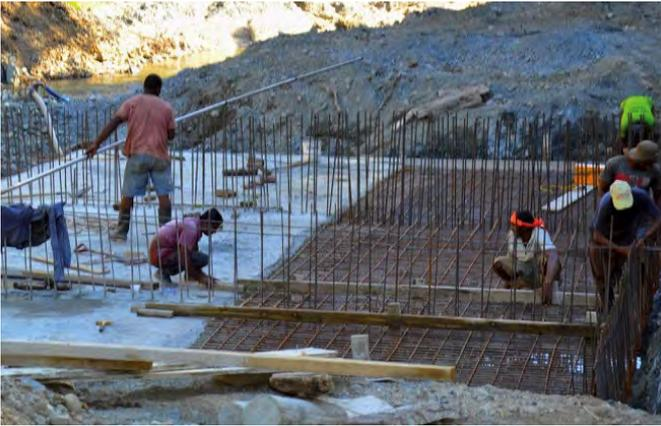
Photo: Retaining weir to prevent flooding that is under construction in Nadi, Fiji (SDC).
