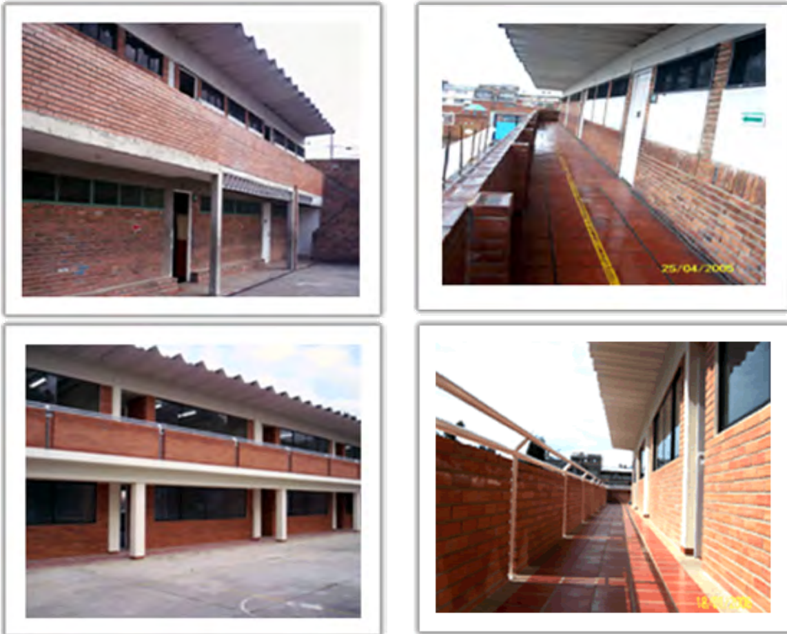
Figure 4. Structural reinforcement and other interventions of a school to improve security
