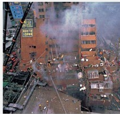
Ruined residential Building
