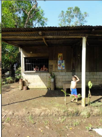
House located in a high risk flood zone
