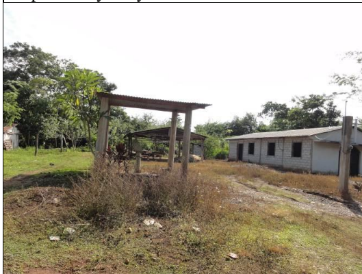
Community water pump
