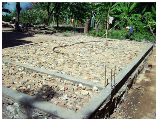
Appendix Figure 3. A closed foundation of a new house found on site
