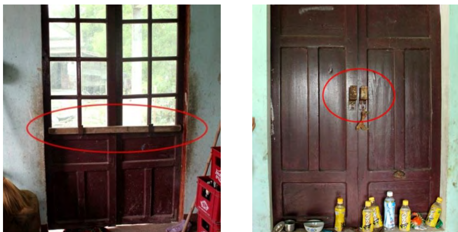
Appendix Figure 7. Strengthening wooden bars for door (left) and window (right) found in a DWF house visited in Loc Vinh
