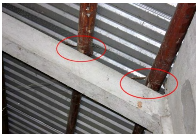
Appendix Figure 6. Strong roof connections in a DWF house visited
