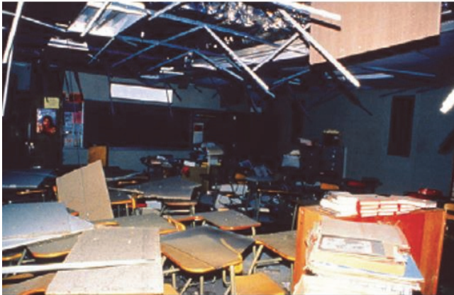
(b) Ceiling damage in a classroom in the 1994 Northridge earthquake.
