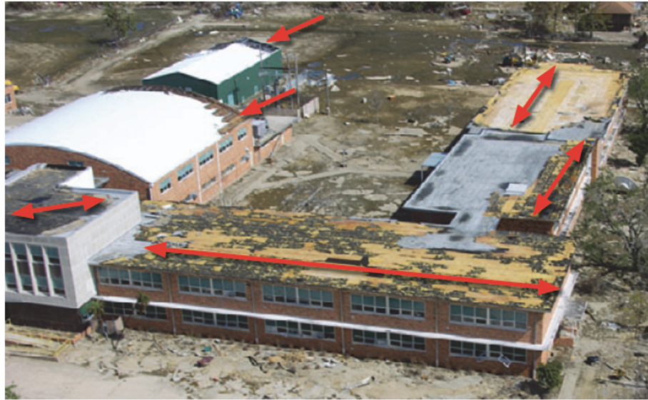
Figure H-3 Large portions of the school roof coverings blew off (indicated by red arrows) during 2005 Hurricane Katrina (FEMA, 2010a).
