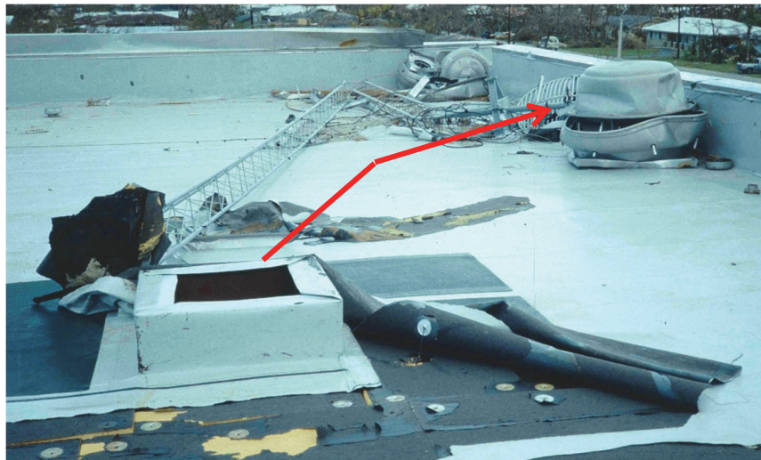
Figure H-14 Rooftop mechanical equipment is often inadequately attached (even on new schools). Several exhaust fans blew off their curbs, allowing rain to directly enter the school during Hurricane Andrew, Florida in 1992. It is very inexpensive to anchor equipment and avoid costly damage (FEMA, 2010a).
