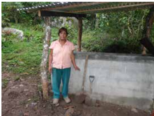
Gisella Hoyes, a producer from the community of El Castillo, benefited from the construction of a demonstration biofilter. (Photo: Nicaraguan Red Cross)
