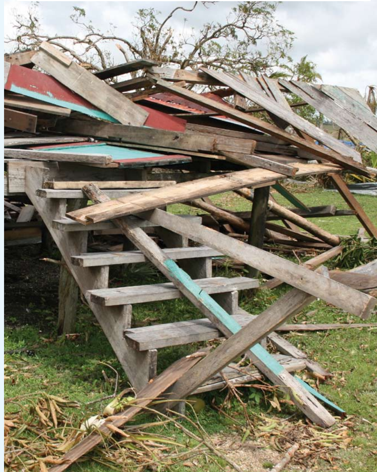
Damage by Hurricane Felix in Krukira, Nicaragua. Virtually everything built of wood collapsed. The few buildings left intact were concrete. Photo: Alex Wynter/International Federation of Red Cross and Red Crescent Societies
