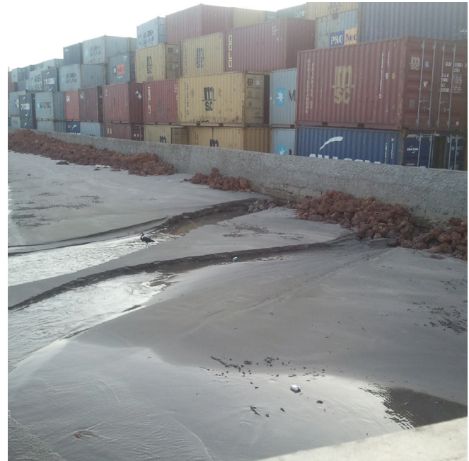
Figure 3. Gambia: the beach is squeezed between development and the sea, unable to retreat, the beach lowers and protection is lost
