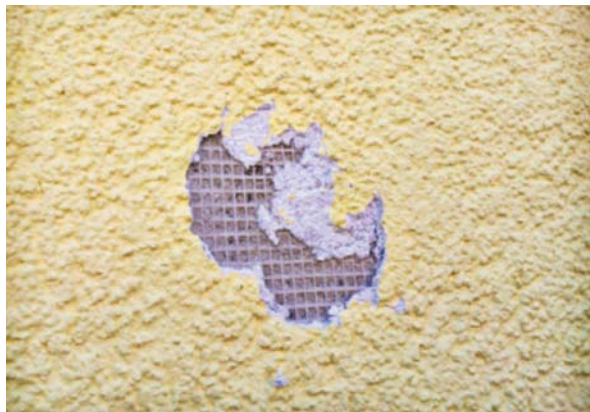
Newer, well-insulated façades with a thin finishing coat proved to be very susceptible to hail damage.
