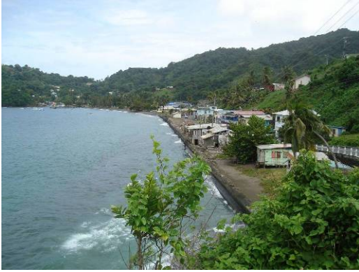
Tyrrels Bay Speyside bay south sea wall
