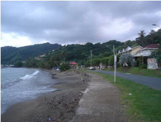
Coastal sea wall along the Speyside Bay Windward Main
