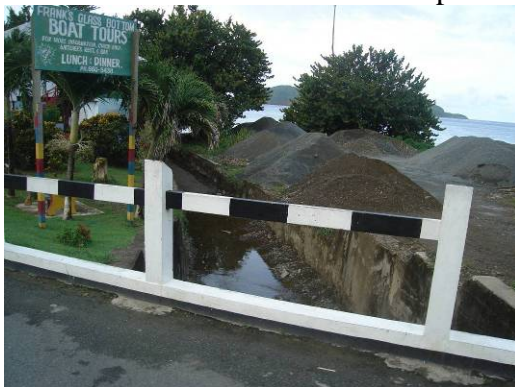
Examples paved drainage channels within Speyside Village
