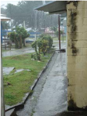
Example of the village conditions during a rain storm Note the full capacity of the drainage (Government Housing Settlement Scheme)
