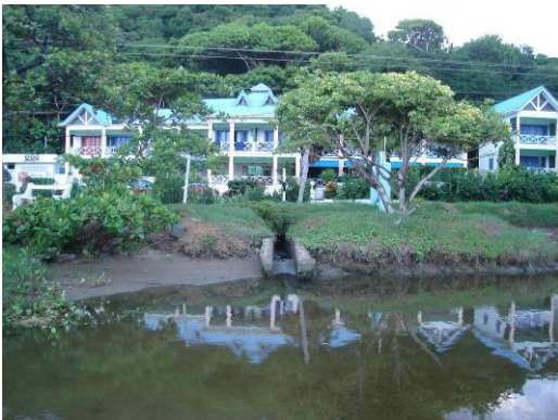
Drainage waste outfall for the road and hotel on into Doctor River mouth on Speyside bay
