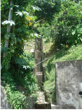
Example of steep hillside drainage (Top Hill Village) Note the steep slope of the drainage System,
