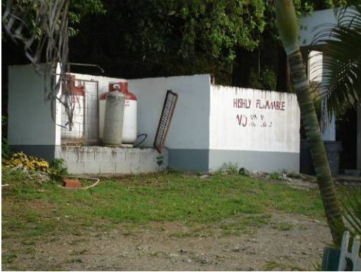
Example of a commercial operation with poor LNG storage controls. Mata Lodge Hotel
