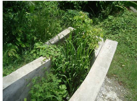
Example of a poorly designed flood drain which can pose a hazard
