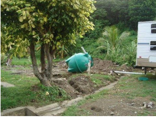
Example of a private sewage Septic tank in installation process
