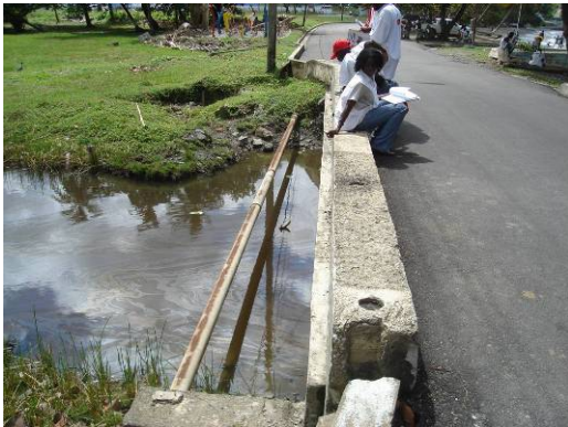
Lucy Vale Beach or Trios Rivieres Beach (Tyrrels Bay) wetland Note drainage water line and road way bridge which on the beach side can block drainage flow
