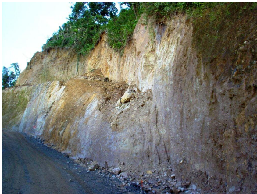
Road works taking place in area prone to landslide
