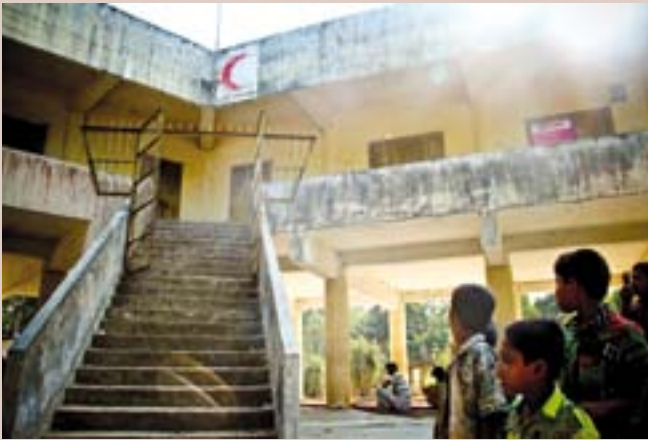
Shelter built by the Bangladesh Red Crescent Society in Cox’s Bazar where BRAC has set up a primary school. ©Himadri Ahsan/BDRCS.
