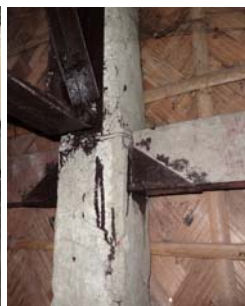
Above: IFRC SRU Shelter Solutions Bangladesh: improved connections
