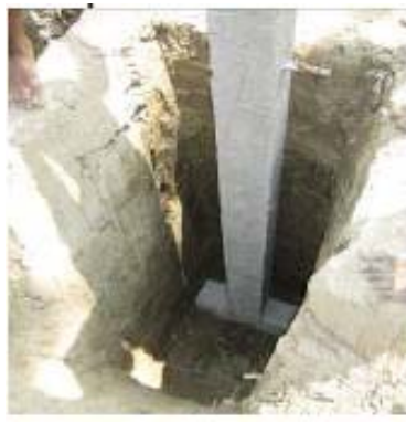
Above: IFRC SRU Shelter Solutions Bangladesh: different types of reinforced concrete foundations
