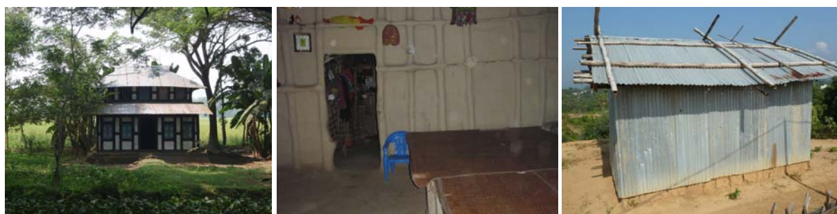
Above: Friendship – IFRC SRU fieldwork conducted in Fall 2015: examples of local construction techniques, from left to right: Kalapara panel housing, Sylhet wattle and daub, Rangamati tribal housing
