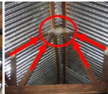
Above: IFRC SRU Shelter Solutions Bangladesh: tie down from bottom to top
