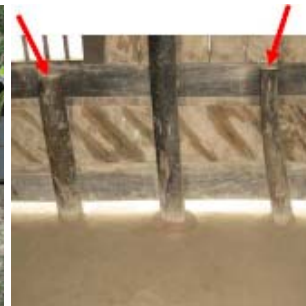
Above: IFRC SRU Shelter Solutions Bangladesh: tie down from bottom to top
