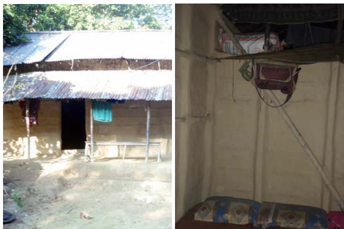
Above: Friendship – IFRC SRU fieldwork conducted in Fall 2015, Sylhet: introduction of cross-bracing into traditional wattle and daub construction
