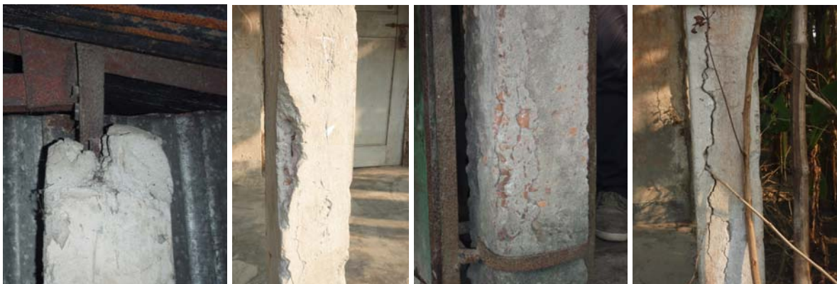
Above: Friendship – IFRC SRU fieldwork conducted in Fall 2015, Kalapara: common problems with reinforced concrete
