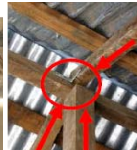
Above: IFRC SRU Shelter Solutions Bangladesh: tie down from bottom to top
