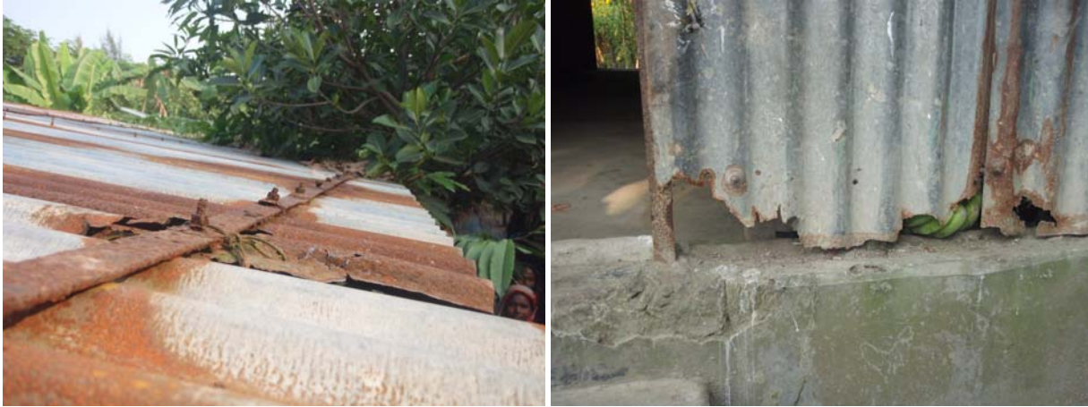
Above: Friendship – IFRC SRU fieldwork conducted in Fall 2015, Kalapara: tin sheets corrode due to lack substandard application
