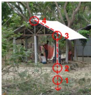
Above: IFRC SRU Shelter Solutions Bangladesh: tie down from bottom to top
