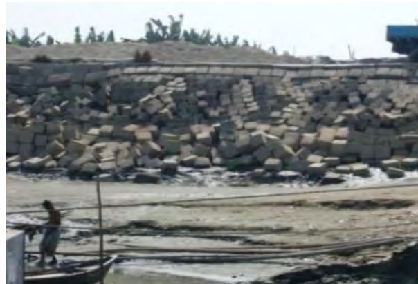
Concrete slope-stabilization blocks
