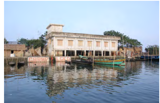
Protection with retaining wall
