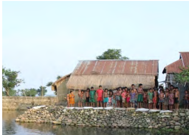
Protection with retaining walls and stones
