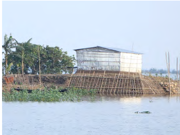
Protection with local stone and bamboo
