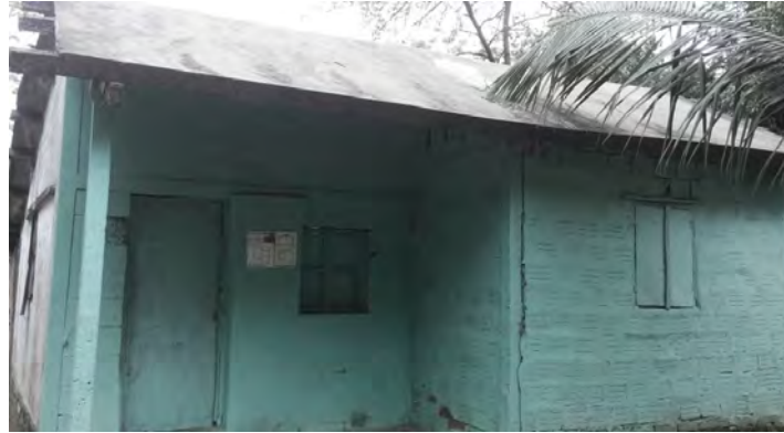
Cast in-situ Ferrocement Roof
