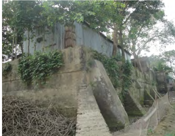
Protection with retaining walls along with buttresses
