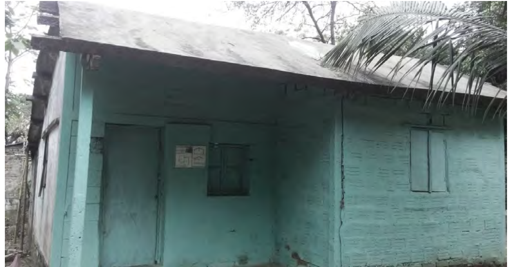
Cast in-situ Ferrocement Roof
