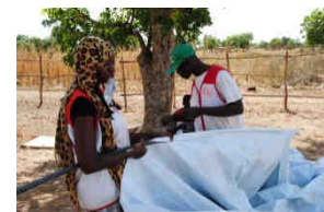
Dome Cladding - Outer Layer
