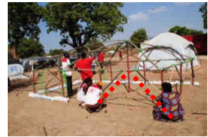
Dome structure and vertical bracing
