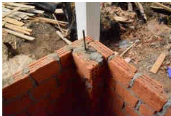
Reinforced angle on interior wall
