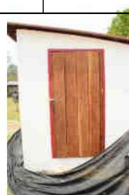
Exterior view with door and walls with plaster and painted
