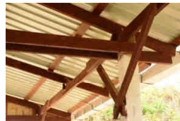
External beam with piece missing
