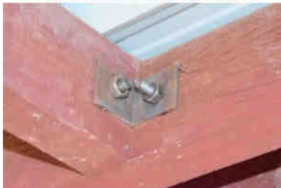
Reinforced joint with metallic angle and bolt Joint angle, exterior view
