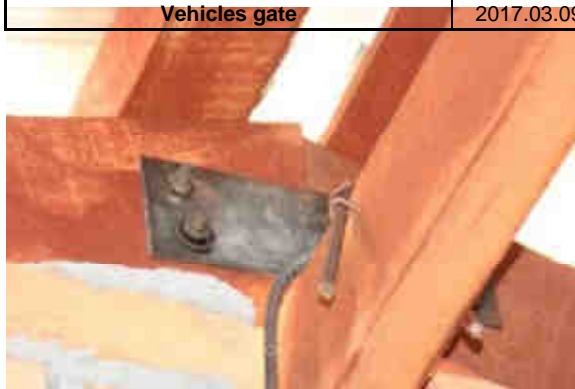
Junction with metallic plate and bolt
