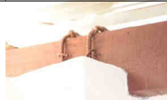
Junction between roof structure and pillar
