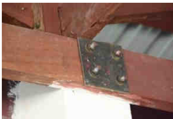
Bolts and metallic plate- joint over pillar
