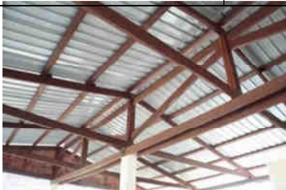
Roof structure with bracing in 2 directions
