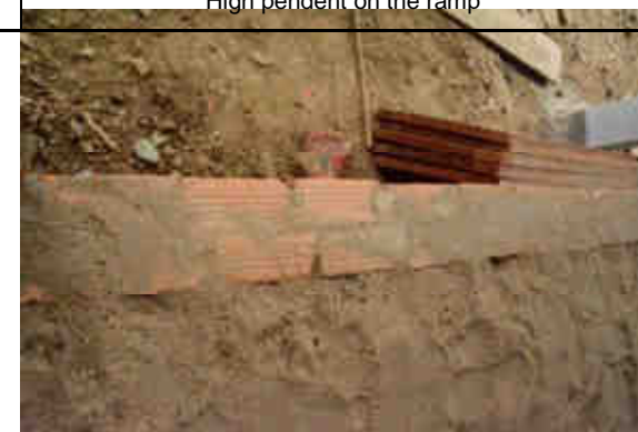
Perimeter wall in 2 layers
