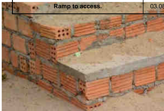
Stairs with brick and concrete slap
