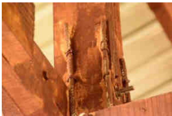
Metallic plate missing over the pillar
