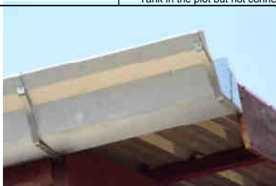
Metallic Gutter
