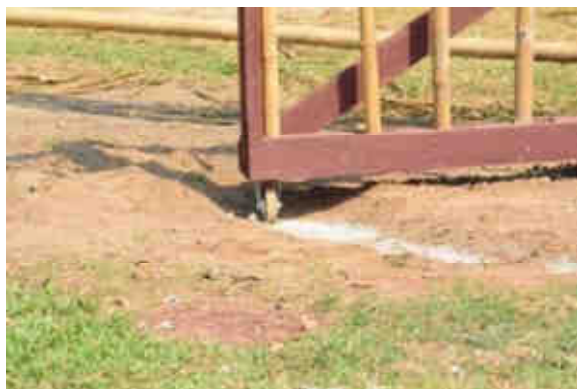
Fence door detail with wheel
