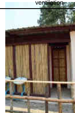
Front view with Bamboo wall and door
