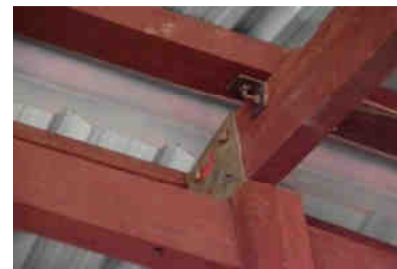
Bolt + metallic plate and L Dephile under the
