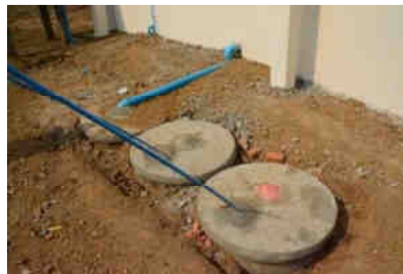
Filtrating pit with ventilation
