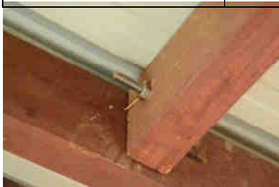
Roof structure joint with bolt and metallic plate
