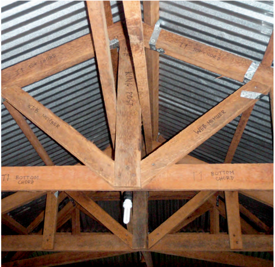
Philippines: Coco lumber roof structure. (IFRC-SRU)
