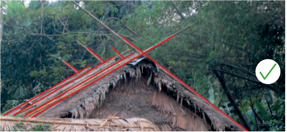
Vietnam, cyclone Nari, 2013: Bamboo placed over the roof covering to prevent it from lifting.
