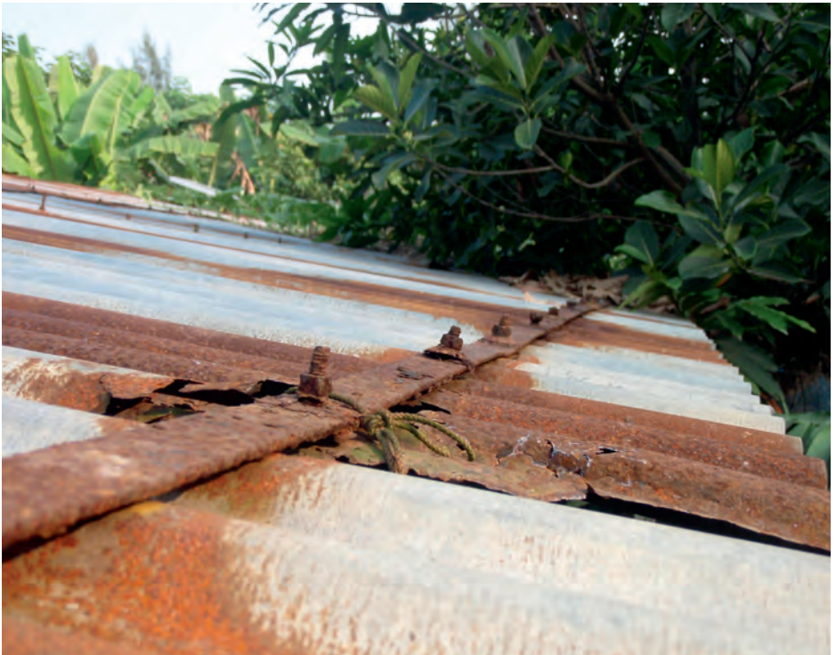
Galvanic corrosion of metall straps and bolts. (IFRC-SRU)
