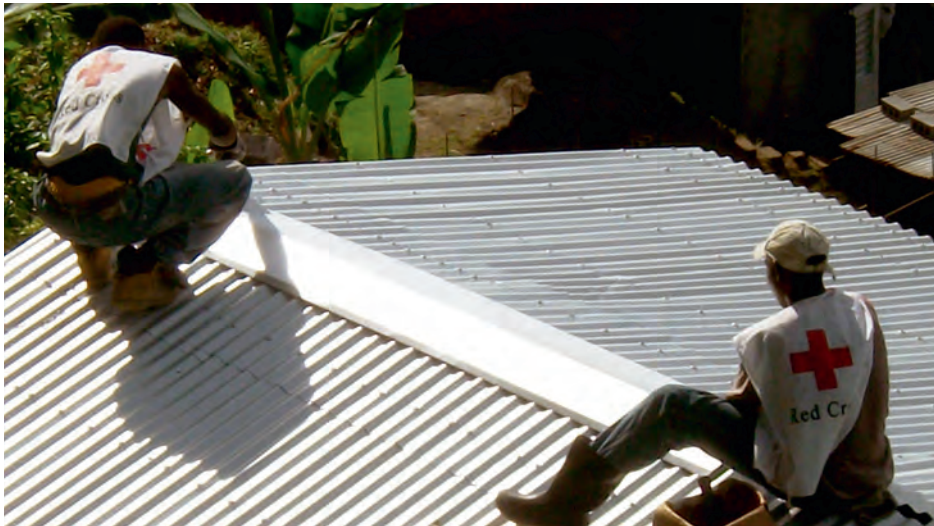
St Vincent & Grenadines, hurricane Tomas, 2010: RC volunteers nailing a ridge cap. (© French Red Cross)
