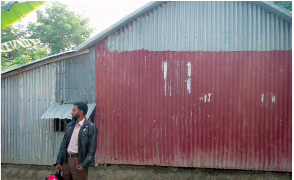
Coastal area Kuakata, Bangladesh: Anti-corrosion-paint used to protect CGI sheets from corroding, especially in marine environment. (IFRC-SRU)
