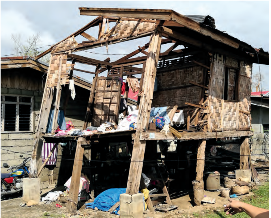
Philippines: Skewed building after typhoon Haima, 2016. (see racking effect on p. 133). (IFRC-SRU)
