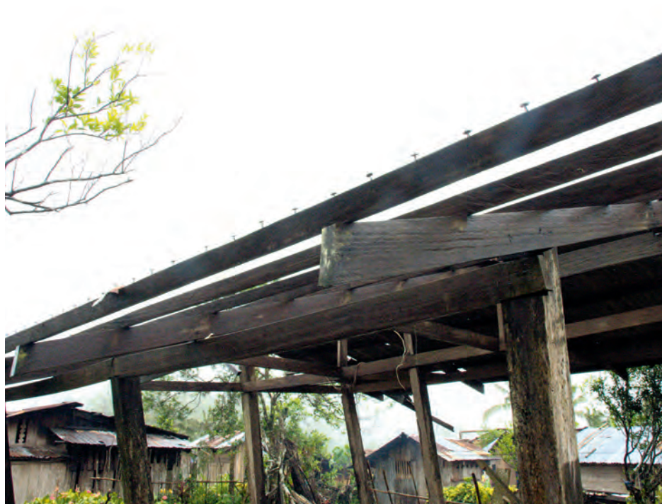
Philippines: Roof structure after CGI sheets unbuttoned. (IFRC-SRU)
