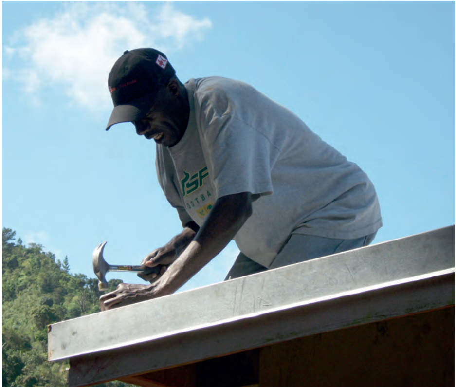
Jamaica: Installation of fascia cap over fascia board. (© French Red Cross)
