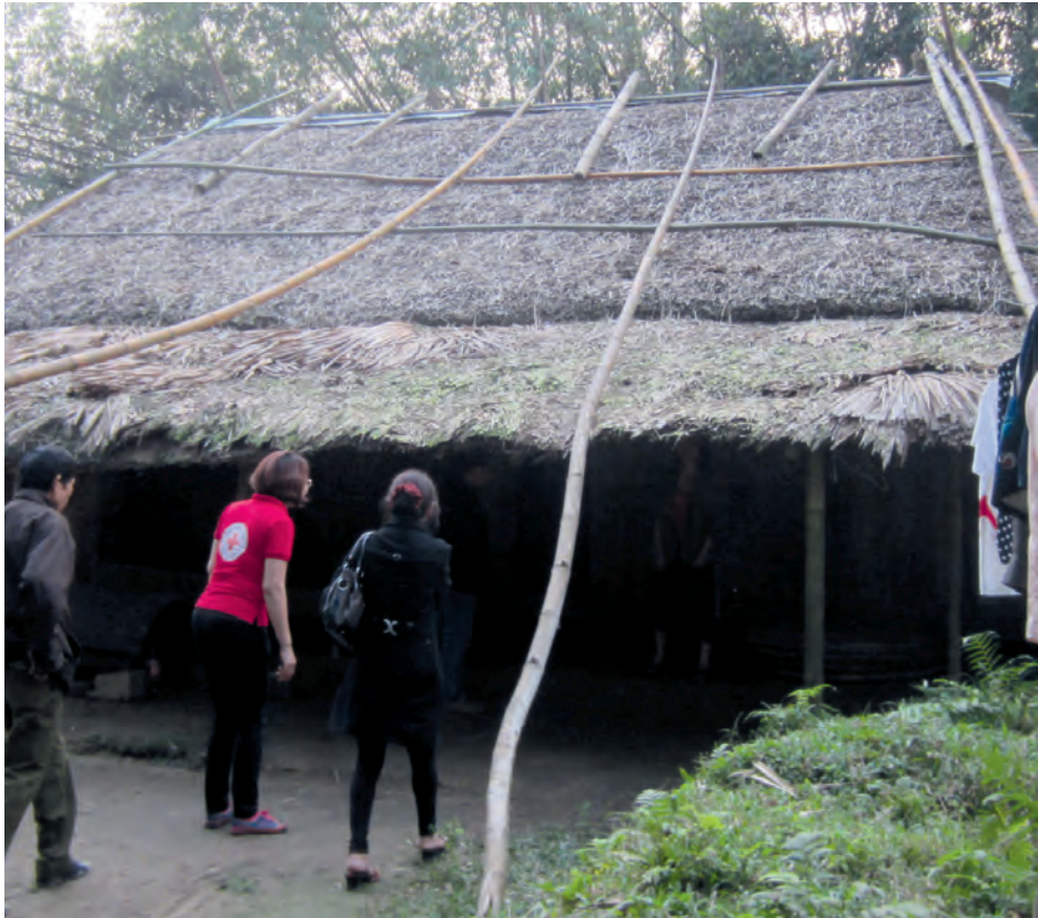
Vietnam, cyclone Nari, 2013: Bamboo placed over the roof covering to hold it down. (© Shelter over head)
