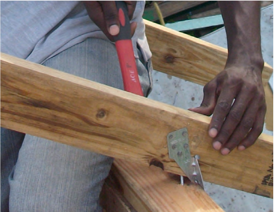
RC volunteer installing a hurricane strap between rafter and wall plate. (© French Red Cross)
