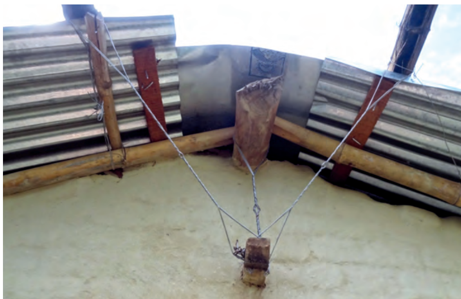
Improvised tie-downs with wire to secure CGI sheets and ridge beam to the wall. (IFRC-SRU)
