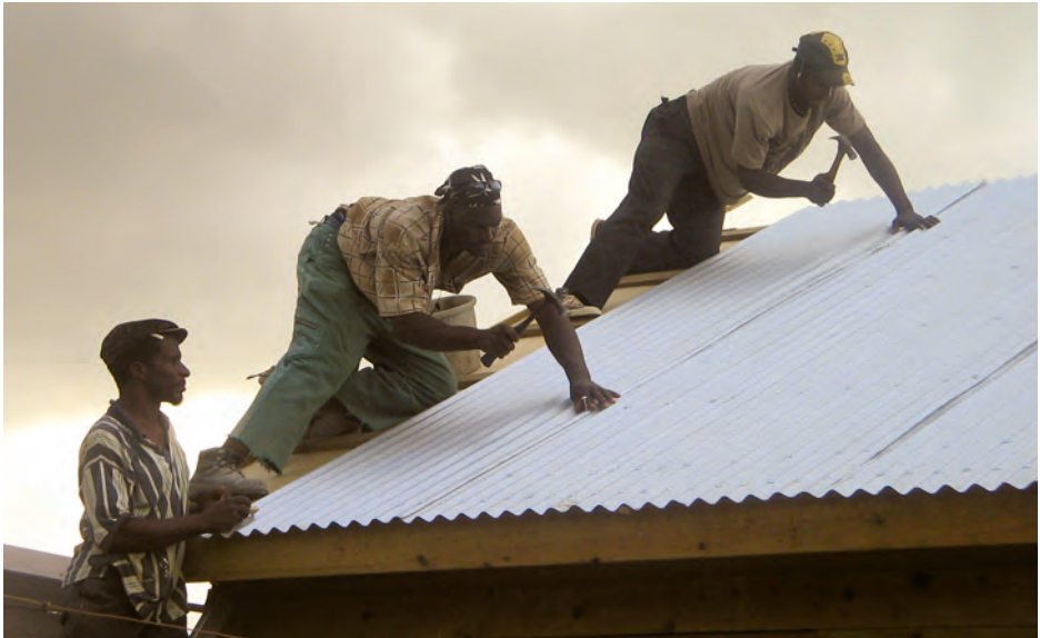
Jamaica, Hurricane Dean, 2007: Builders covering a roof with CGI sheets. (© French Red Cross)
