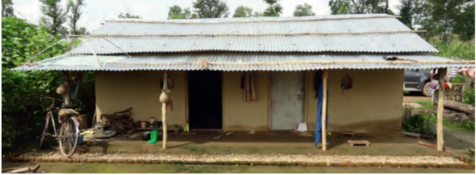
Veranda roof separate from main structure.
