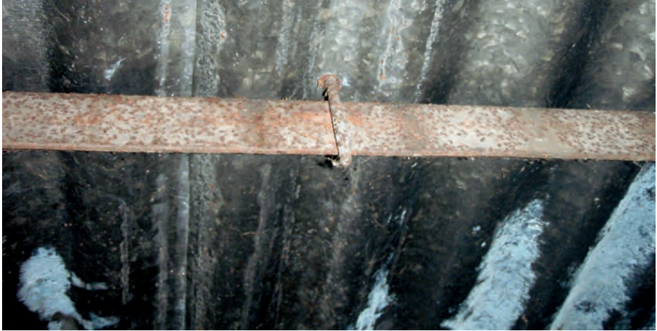
Corroded steel truss and CGI with white rust. (IFRC-SRU)
