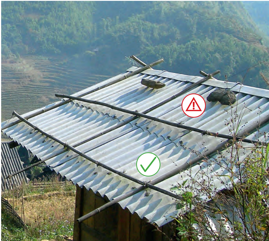
Vietnam, 2006: Bamboo over a gable roof to reinforce it against uplift. Placing stones on the CGI roof is not recommended. (© Netherlands Red Cross)
