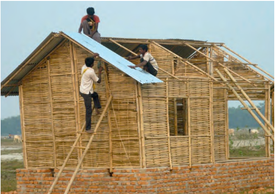
Nepal: Installing CGI on bamboo structure. (IFRC-SRU)
