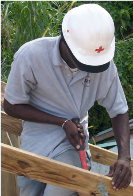
RC volunteer wearing a helmet while installing a hurricane strap. (© French Red Cross)
