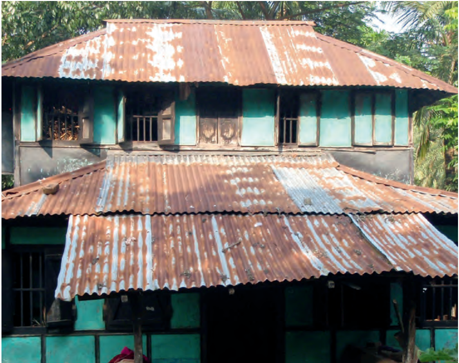
Coastal area Kalapata, Bangladesh: Corroded CGI roofing. (IFRC-SRU)
