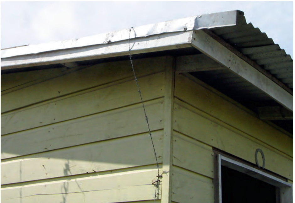
Supports placed over the eaves on a gable roof with different types of anchors
