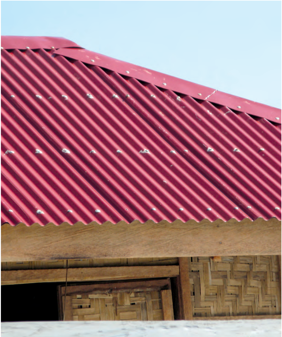
Philippines: Ridge cap and hip caps. (IFRC-SRU)
