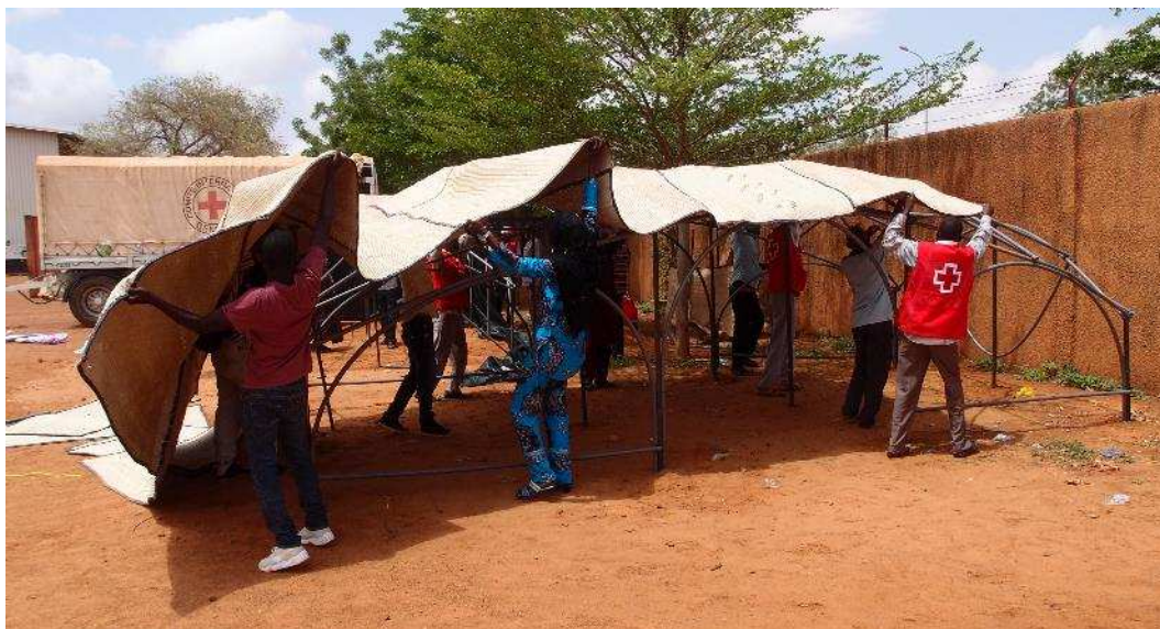
Full cover of vegetal mats for Dome cladding inner-layer
