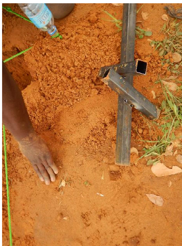
Pole foot with additional pieces for better anchorage
