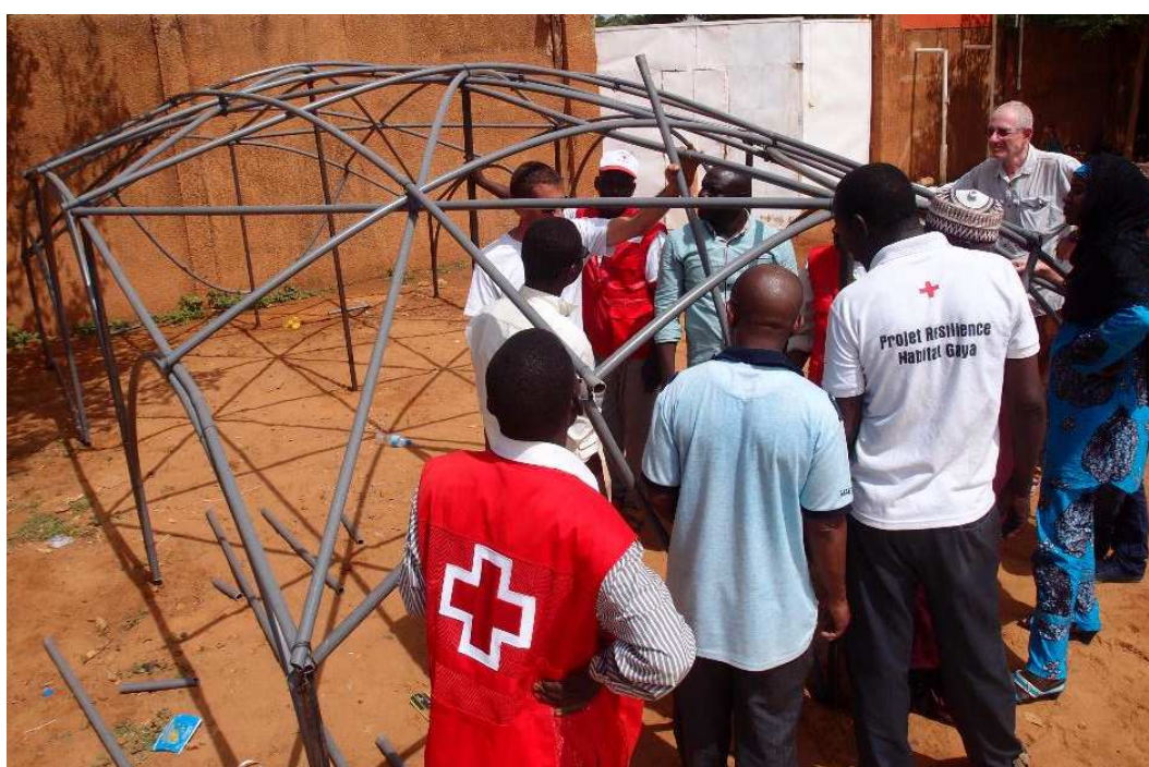
Dome structure with PVC tubes
