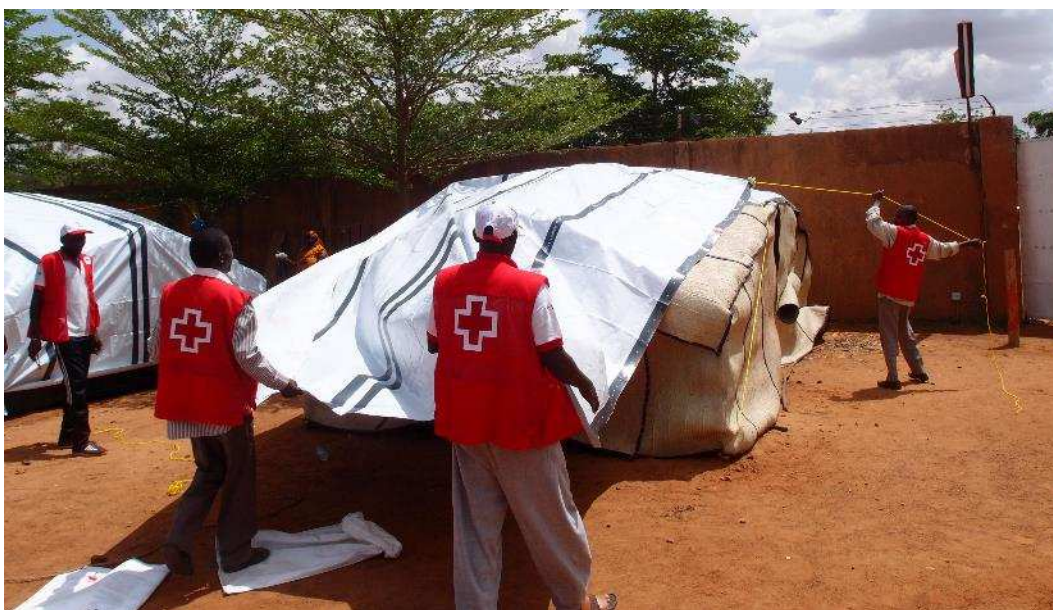
Two IFRC 4x6 tarpaulin for the Dome cladding exterior layer
