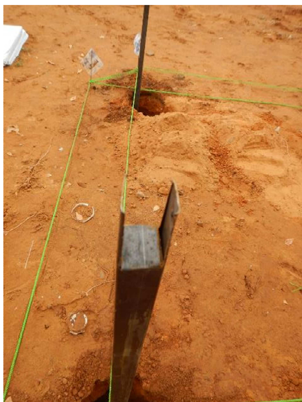
Pole head ready to receive the PVC pipe
