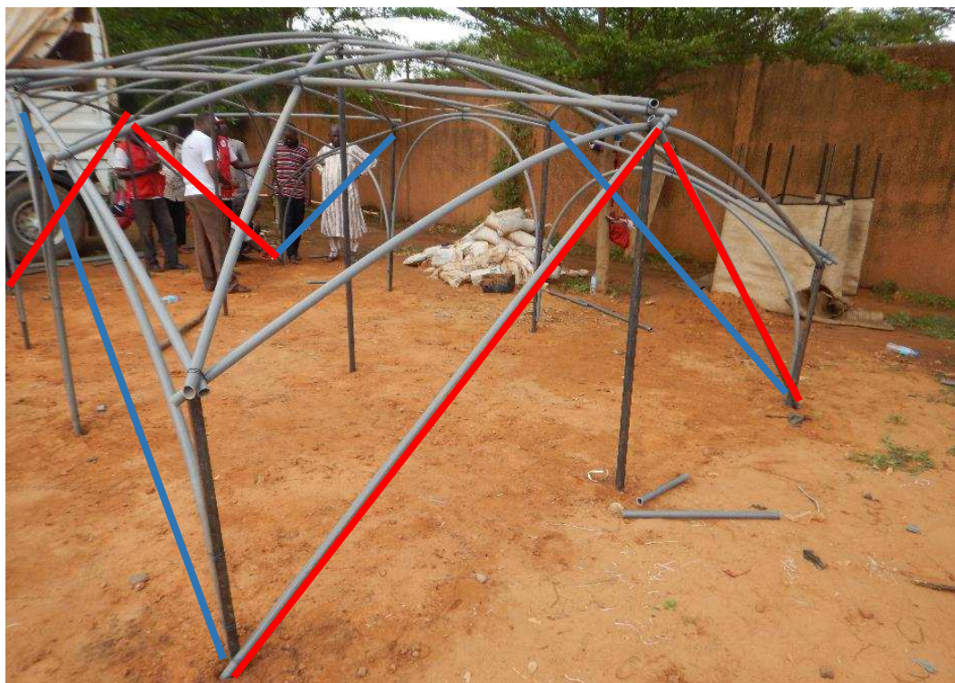
General view of the bracing elements in the two main directions (8 bracings on the walls)
