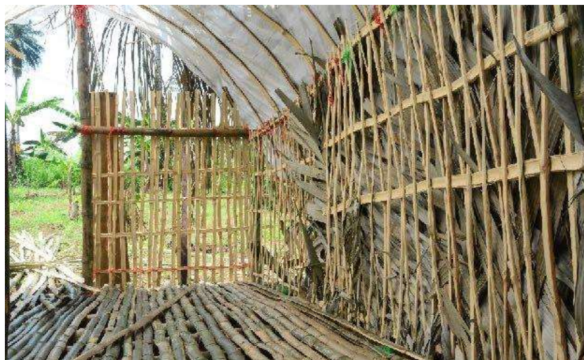
Interior view of wall with bamboo panels during the Edea Workshop
