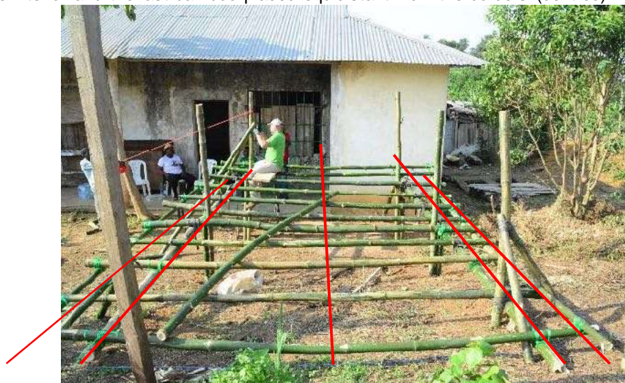
Construction of the semi-rigid platform during Edea workshop
