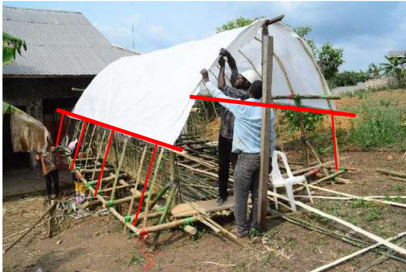
Construction of the first cladding layer over the vault during the Edea Workshop
