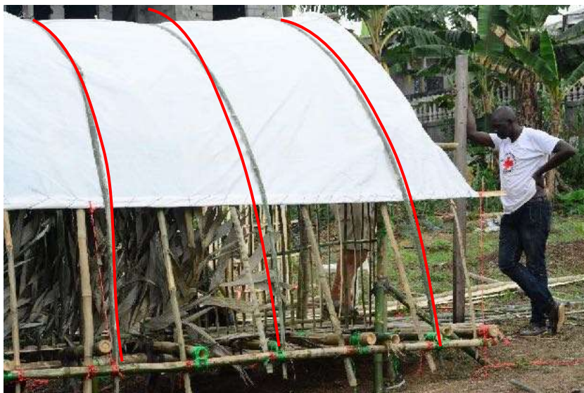
Construction of the second set of bamboo arches over the tarp during the Edea Workshop
