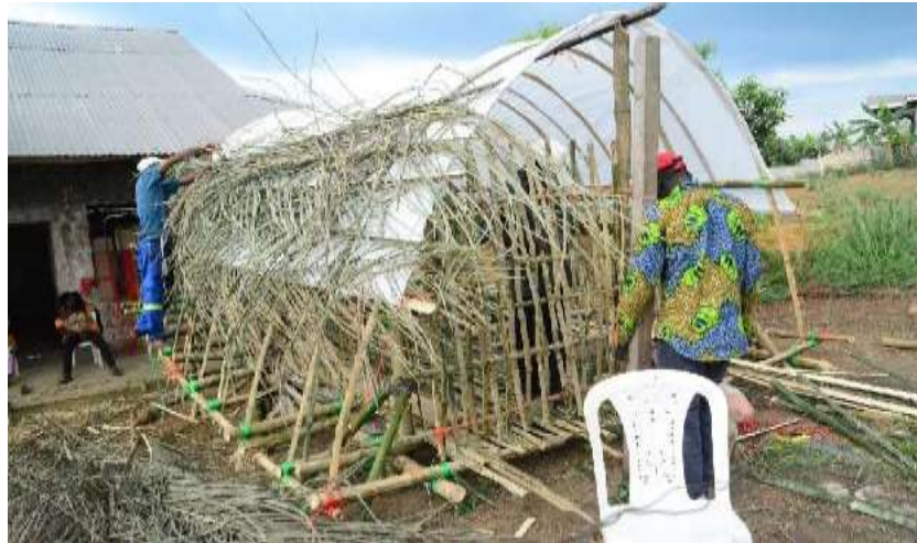
Construction of the second cladding layer over the vault during the Edea Workshop
