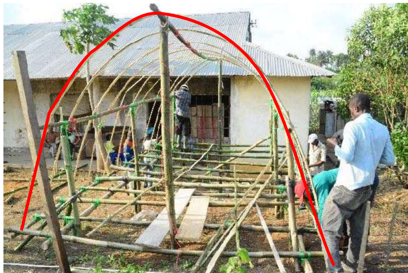
Construction of the vault arches during the Edea Workshop
