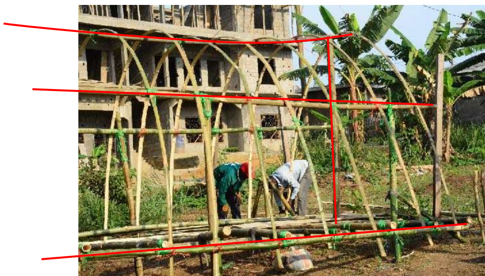
Construction of the vault structure during the Edea Workshop
