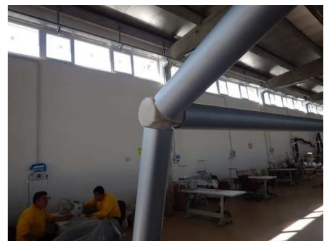
Structure detail- Pipes to plastic joint
