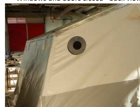
Chimney reinforcement- tent back side
