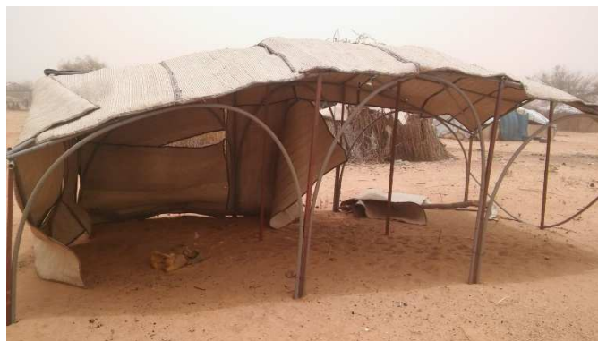
Temporary abanoned Shelter
