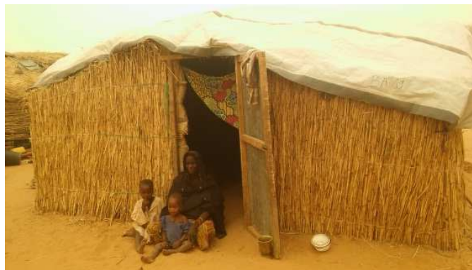
Door with metallic sheet over wood framework
