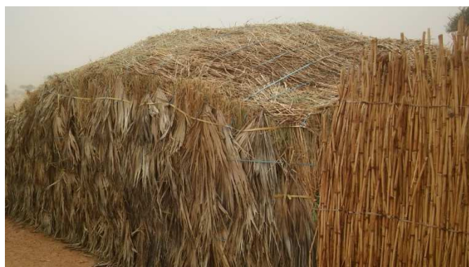
Vegetable layers over the shelter as thermic insulation
