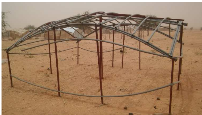
Shelter structure without bracing systems
