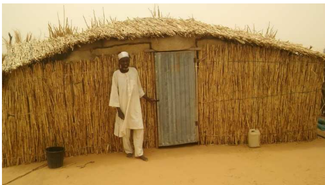
Shelter with modifications in the door and insulation over the roof and walls
