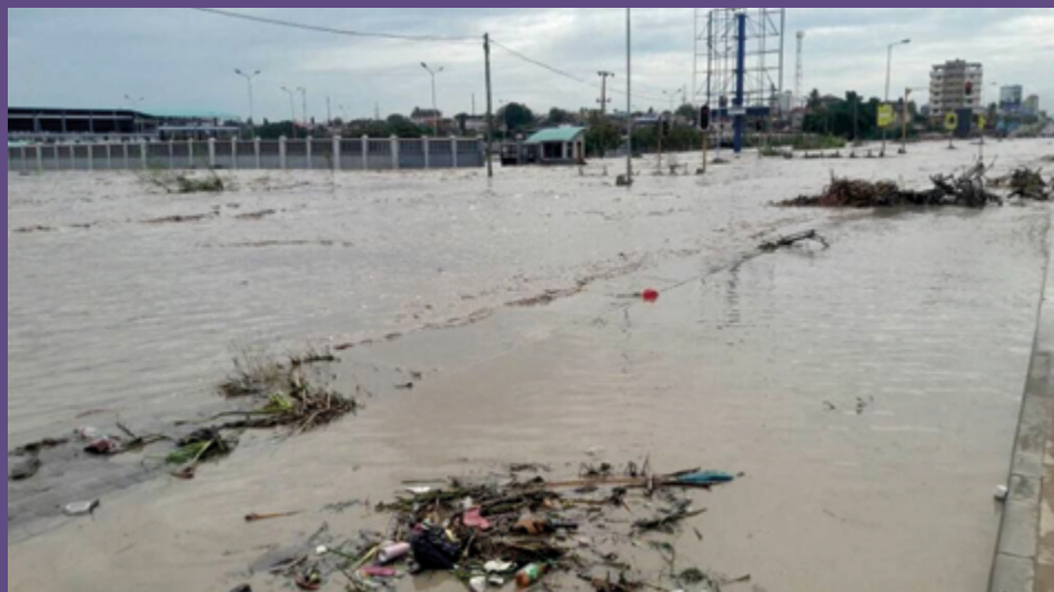
FLOODING AT JANGWANI BRIDGE ON 26 OCTOBER 2017
