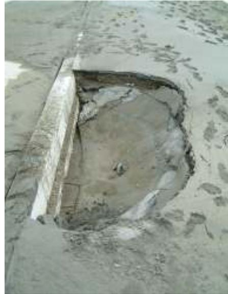
*(2) - Caving due to liquefaction*
