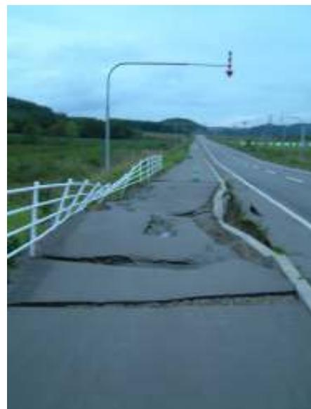
*Photo A3.d - Bank failure*
