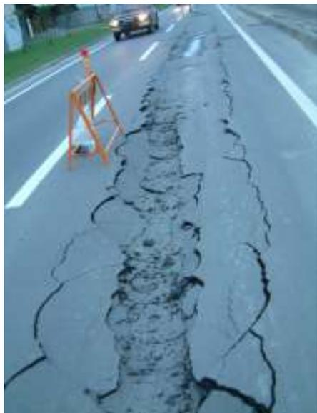
*(3) - Sinkage of backfilling for pipeline*
