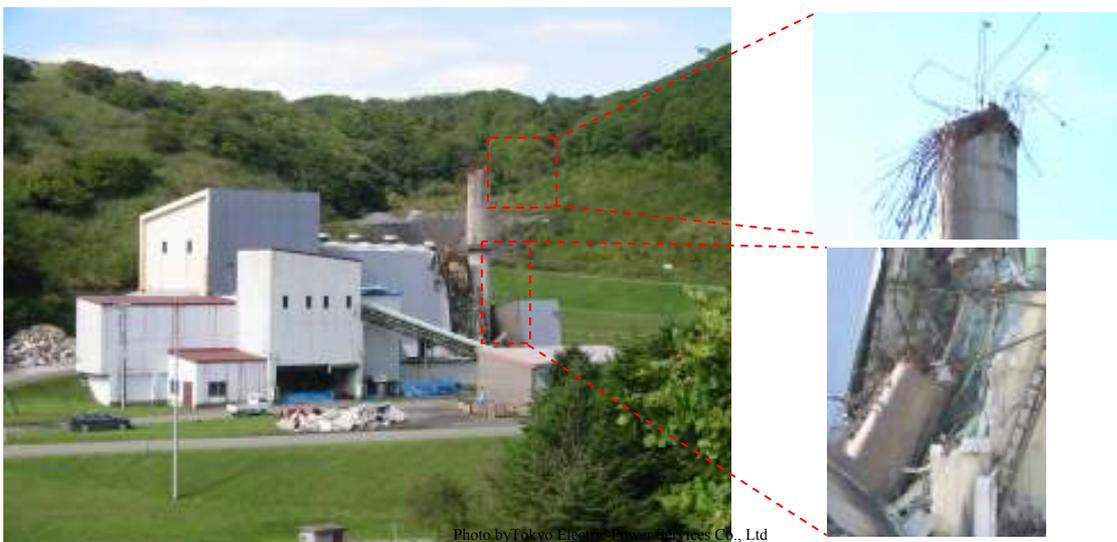
*Photo A3.d - Collapsed chimney of garbage disposal facilities.*
