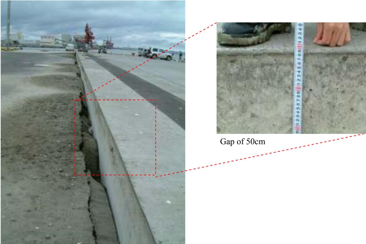
*Photo A3.e - Damage to port facility.*
