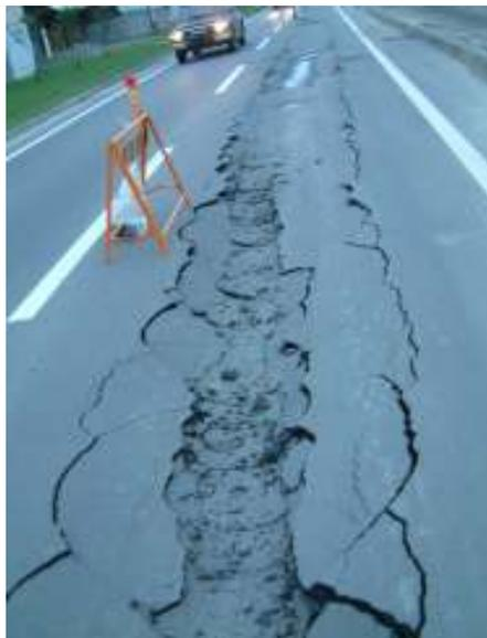
*(3) - Sinkage of backfilling for pipeline*
