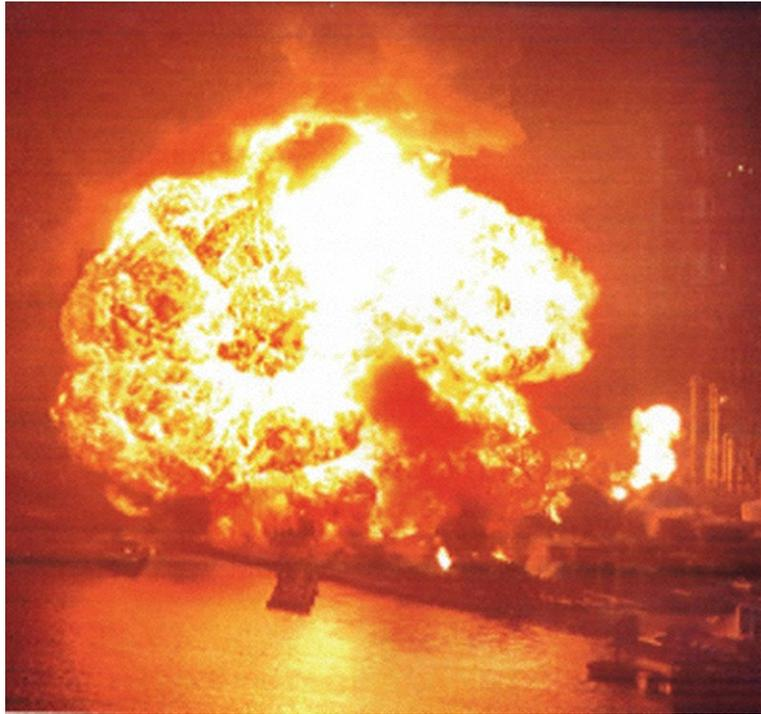
FIGURE 2.4 Fireball at the LPG Storage Farm With a Diameter of About 600 m
