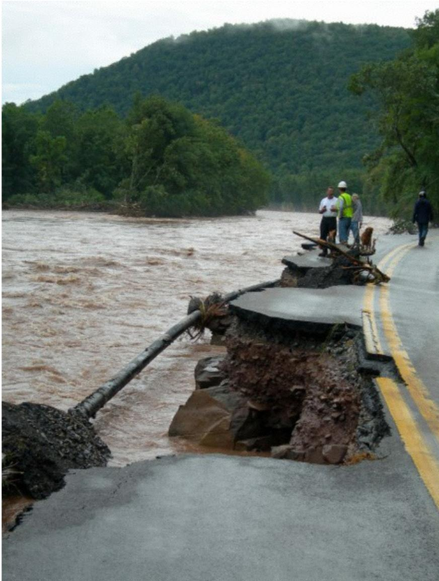
FIGURE 3.5 Exposed Petroleum Pipeline Due to Flooding in Pennsylvania, USA
