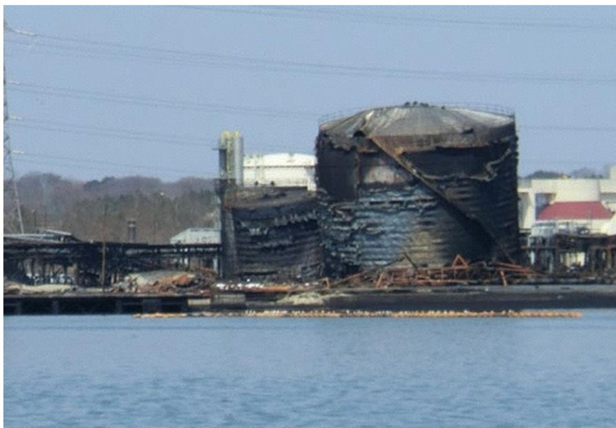
FIGURE 2.6 Burned Tanks at the Sendai Refinery Hit by the Tsunami
