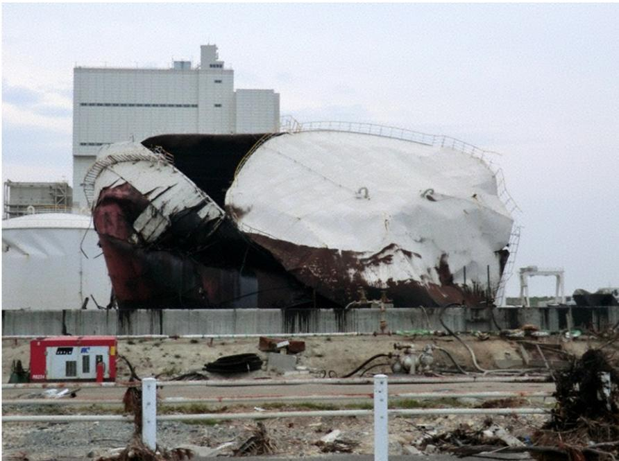
**FIGURE 3.4** Destroyed Heavy Oil Tank at a Thermal Power Plant Battered by the Mega Tsunami in the Wake of the 2011 Tohoku Earthquake in Japan
