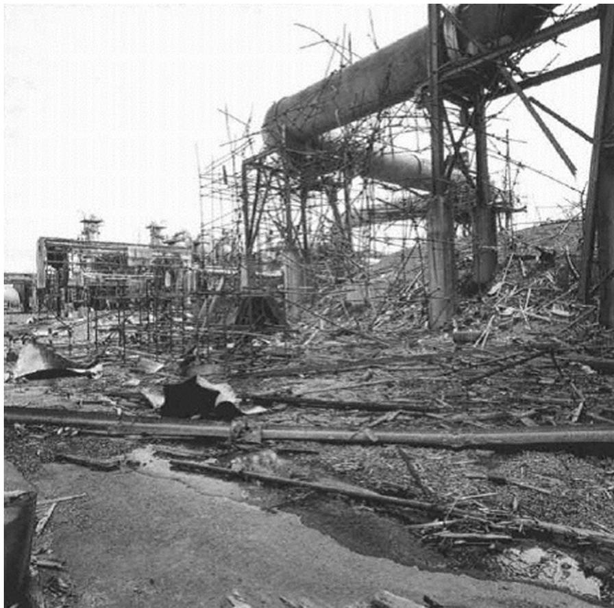
FIGURE 2.10 Major Damage on Site Caused by the Explosion
