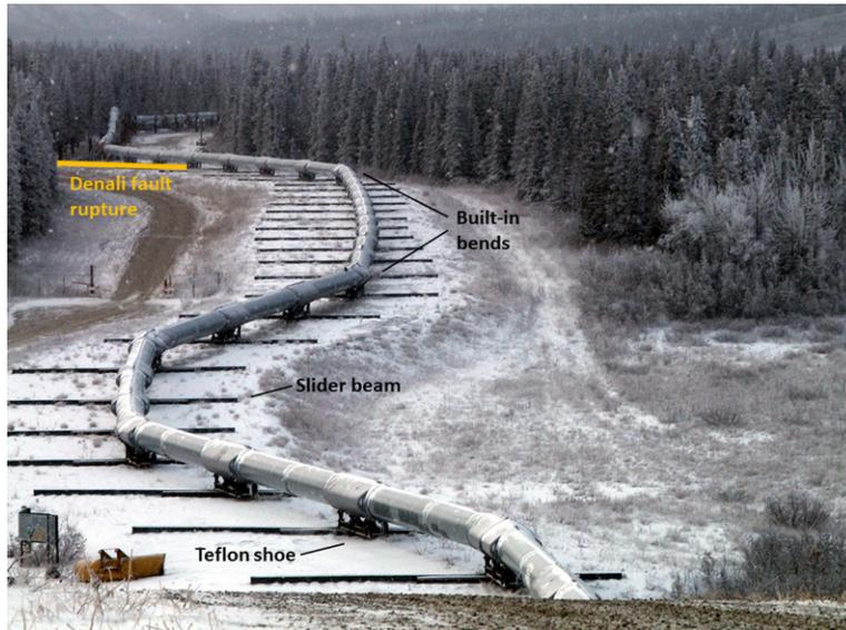
FIGURE 13.3 Engineered Seismic Protection Measures Implemented for the Trans-Alaska Pipeline at the Denali Fault Crossing
