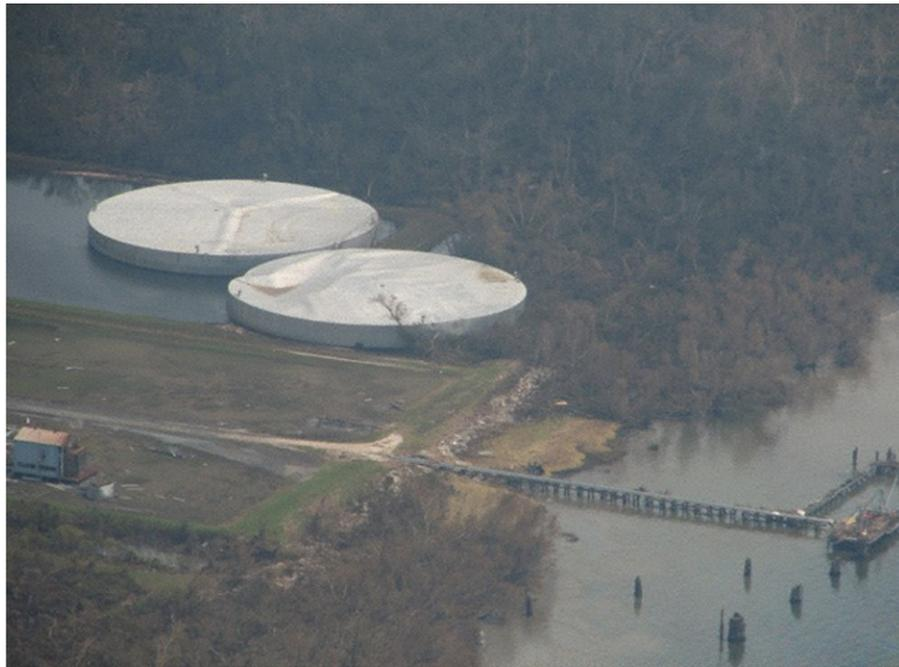
**FIGURE 3.7** The Water and Gale-force Winds Accompanying Hurricane Katrina Floated and Displaced Two Half-Filled Tanks Along the Mississippi River With 3.8 Million Gallons of Oil Pouring From the Tanks
