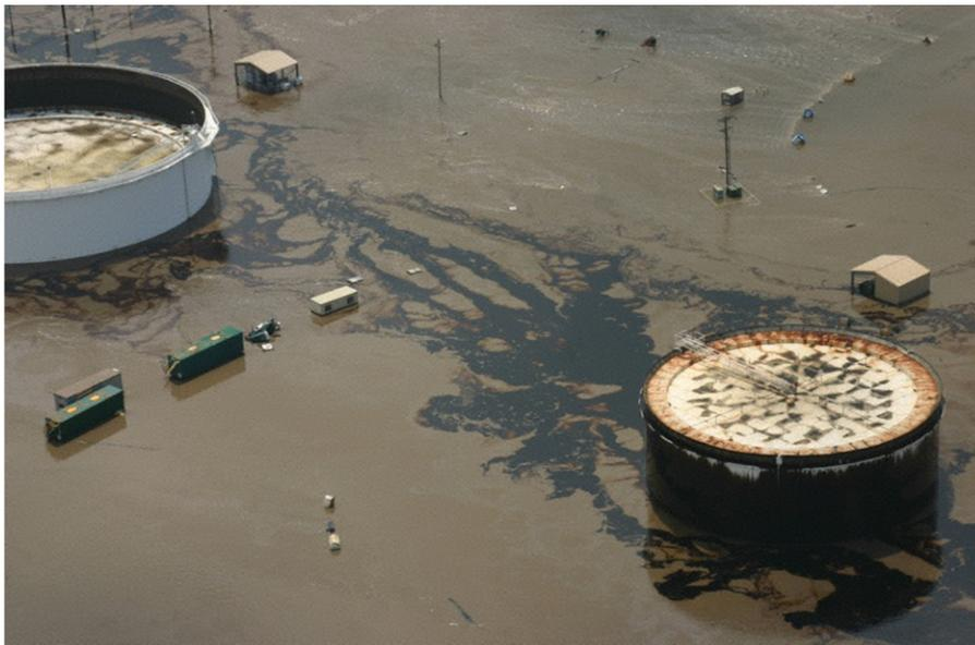
**FIGURE 3.6** Hydrocarbon Release at a Refinery During the Coffeyville Floods in the USA in 2007
