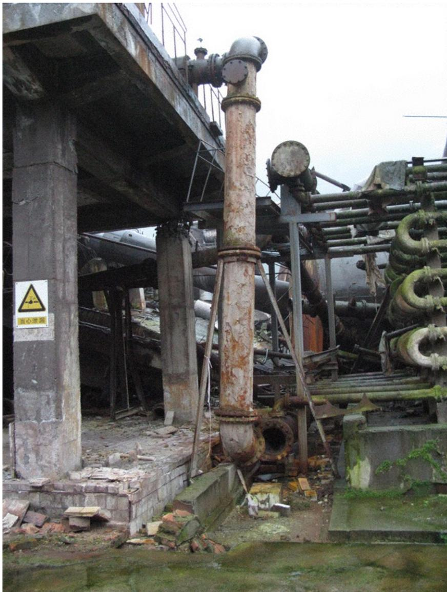
FIGURE 3.3 Flange Failure at a Fertilizer Plant in the Area Hit by the Wenchuan Earthquake
