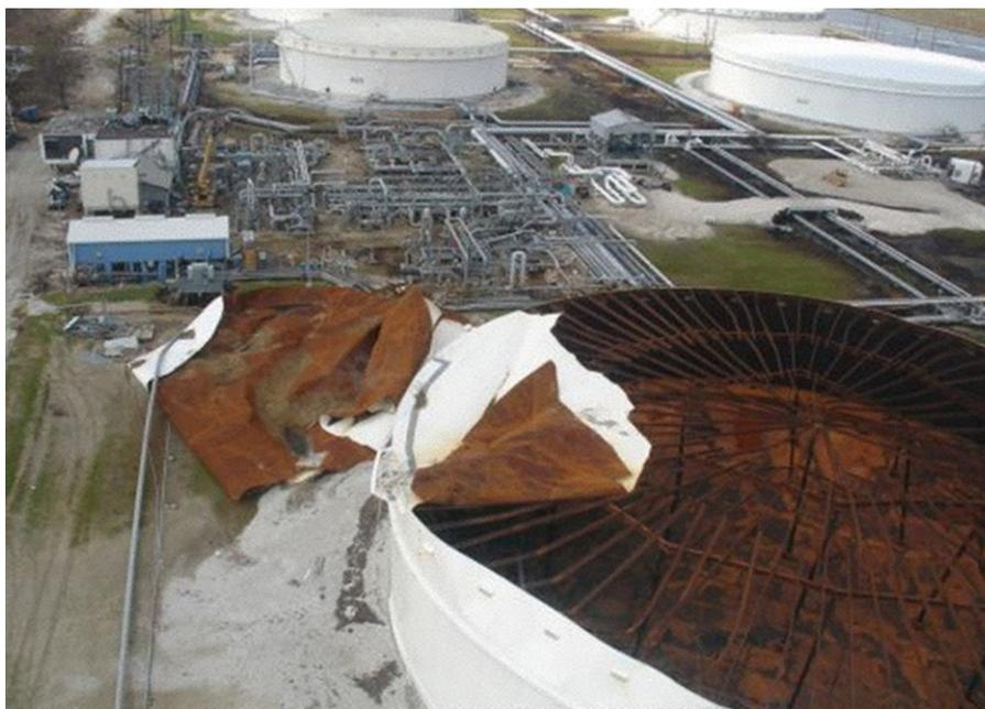
FIGURE 3.8 Wind-Induced Destruction of a Fixed Tank Roof at an Oil Refinery During Hurricane Katrina
