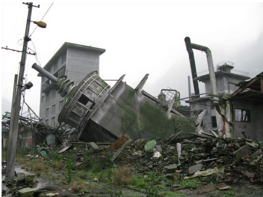
FIGURE 3.2 Collapse of a Dryer and Pipe Severing at a Fertilizer Factory Hit by the 2008 Wenchuan Earthquake in China
