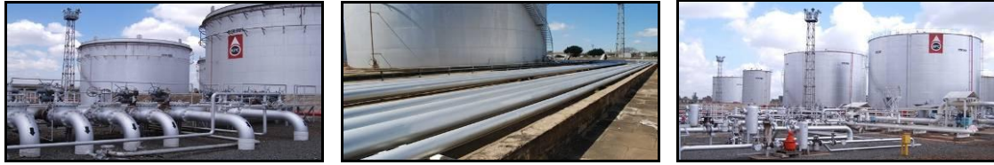
Photography of the KPC petroleum deposit facility - www.kpc.co.ke
