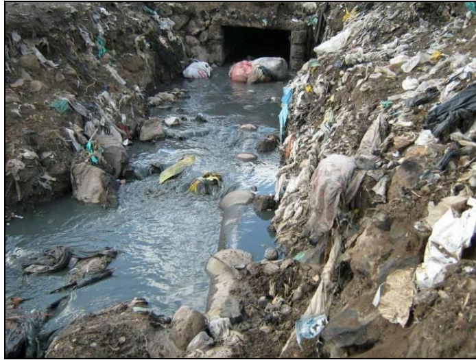
View of the outlet of the storm water drainage network in the slum
