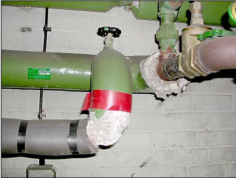
Figure 5 – A comprehensive asbestos survey is required to determine the presence of other, potentially more hazardous, sources of asbestos throughout Shurob. Note that this image is for information purposes only and not taken in Shurob.
