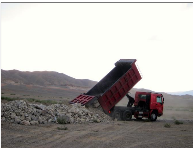
Figure 8 – Construction rubble, from which asbestos has been removed, is used to expand town flood barrier.
