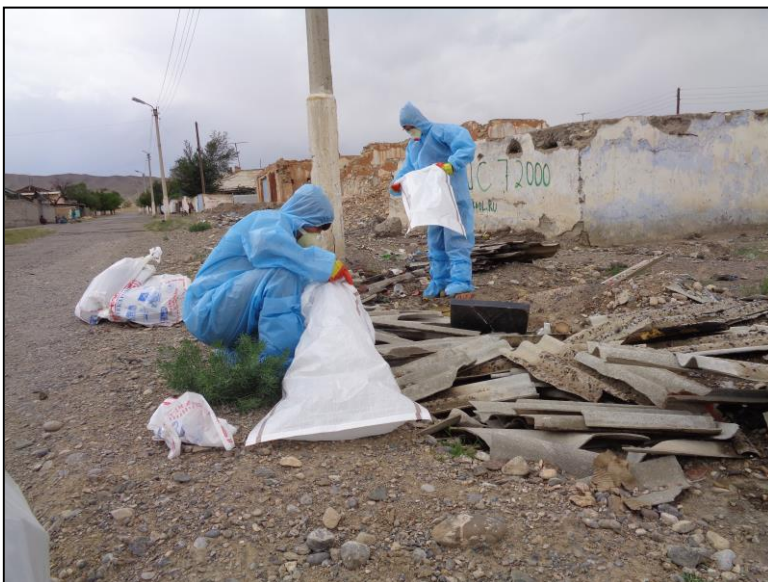
Figure 6 – Participants gained experience in the field of handling, containing and disposing of asbestos waste.
